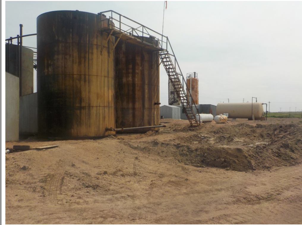
Photo No 3: Description: Dubois Tank Battery facing northeast.
