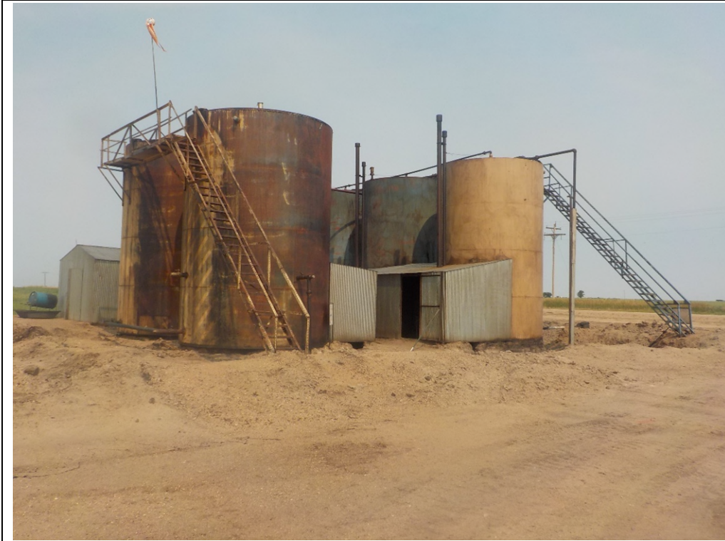
Photo No 4: Description: Dubois Tank Battery facing northwest.
