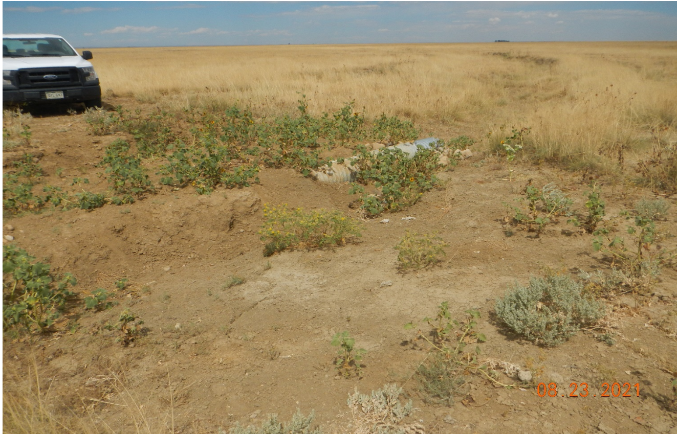
Photo 2. Facing northwest at the drainage crossing that eroded shown in previous photo. This drainage crossing needs to be repaired per good engineering practice.
