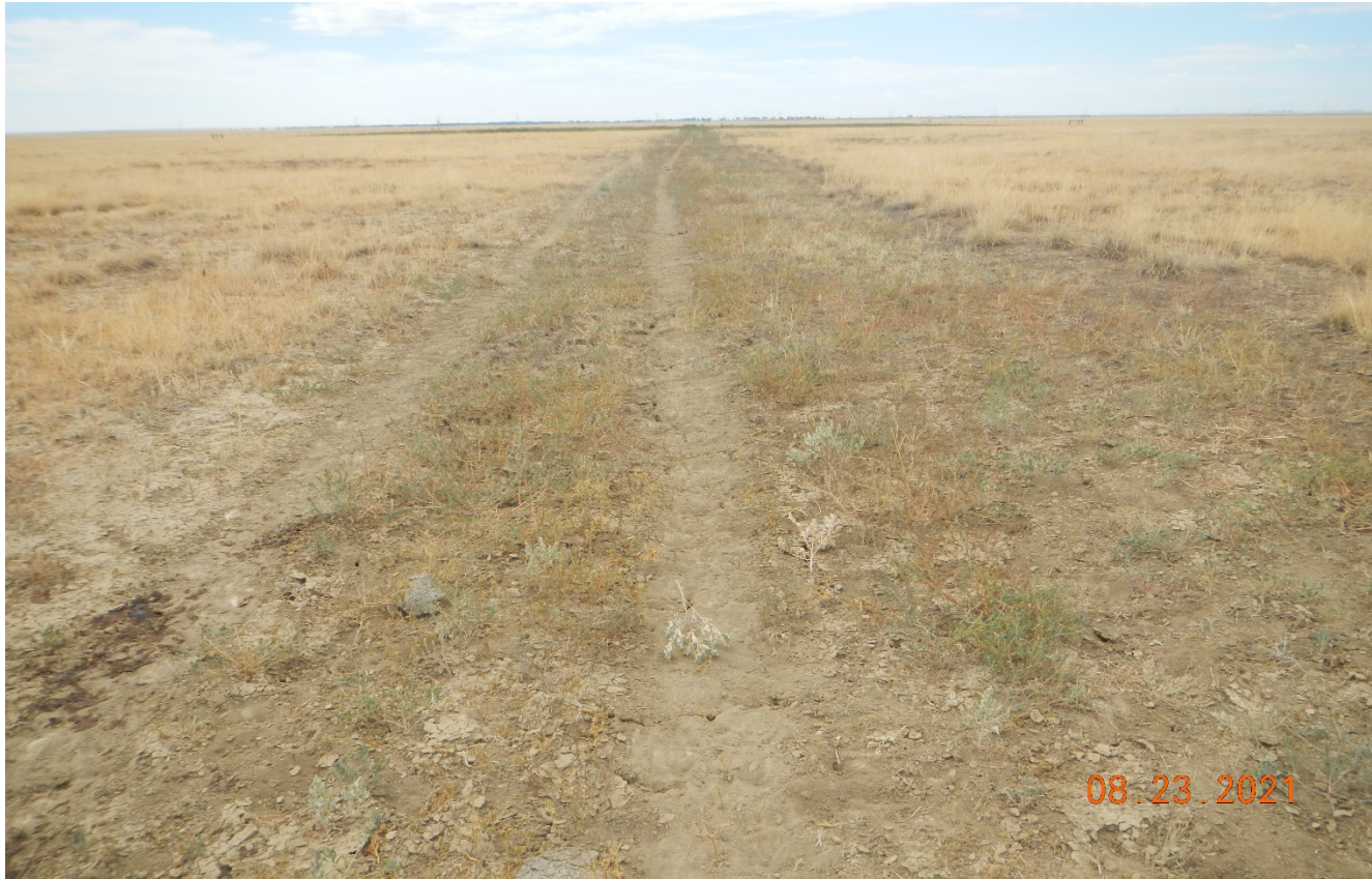
Photo 3. Facing southwest toward the access road which had been reclaimed. The desirable vegetation has failed to establish and will need to be reseeded.
