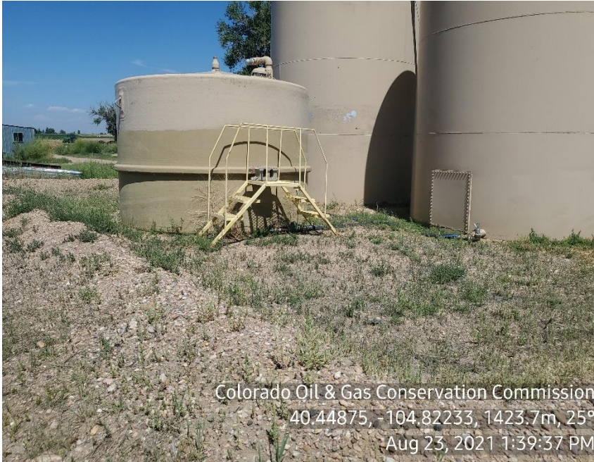
Photo 11: Weeds, inadequate earth berm, no labeling
