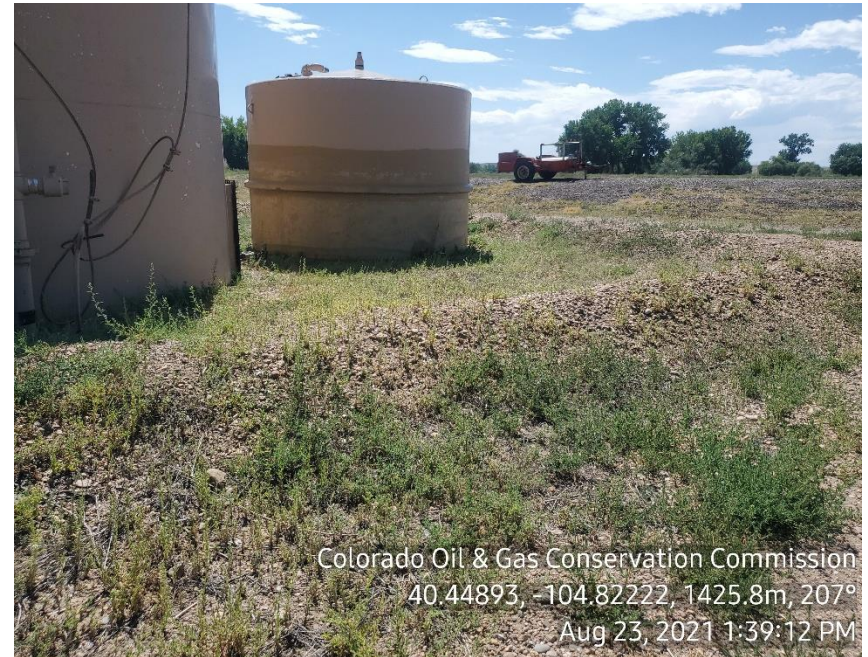
Photo 10: Weeds, inadequate earth berm
