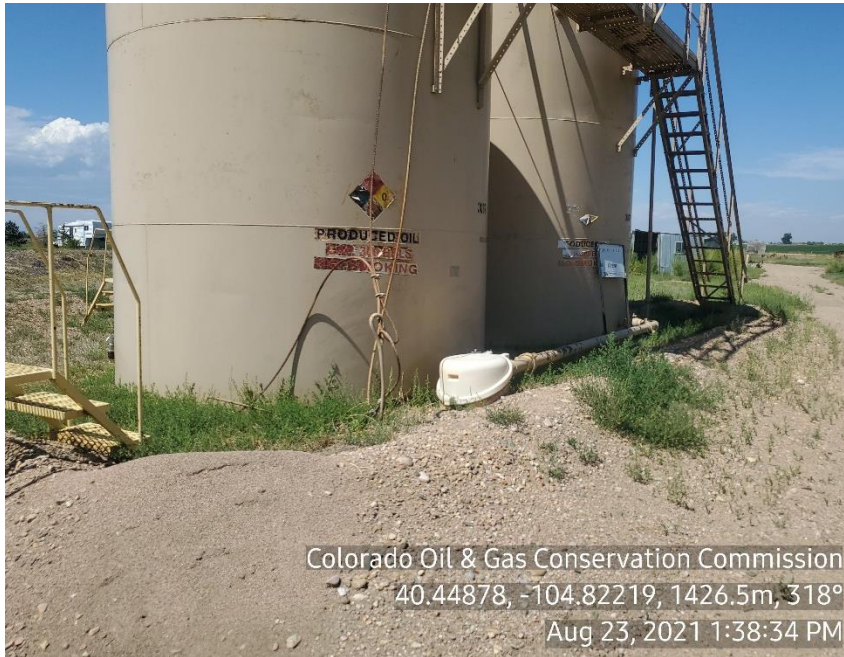
Photo 9: Weeds, inadequate earth berm
