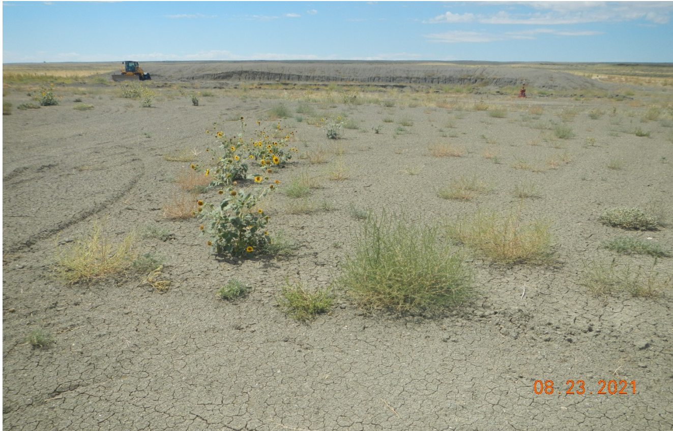
Photo 2. Facing southwest toward the location. Interim reclamation has not been performed. All unused areas of the location need to be reclaimed.
