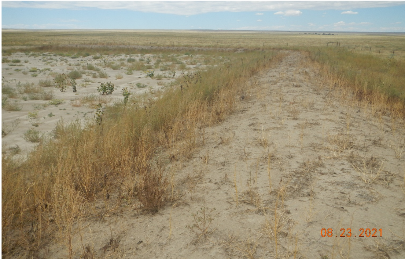
Photo 6. Facing west at the north side of the location. The topsoil pile has not been replaced back to the original position and contour. The topsoil pile is not maintained or stabilized and there are undesirable weeds growing on the segregated soils.
