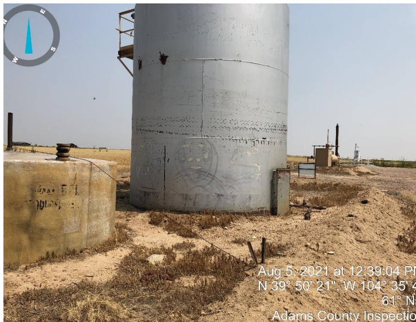
Photo #5 Inadequate berms around tanks.
