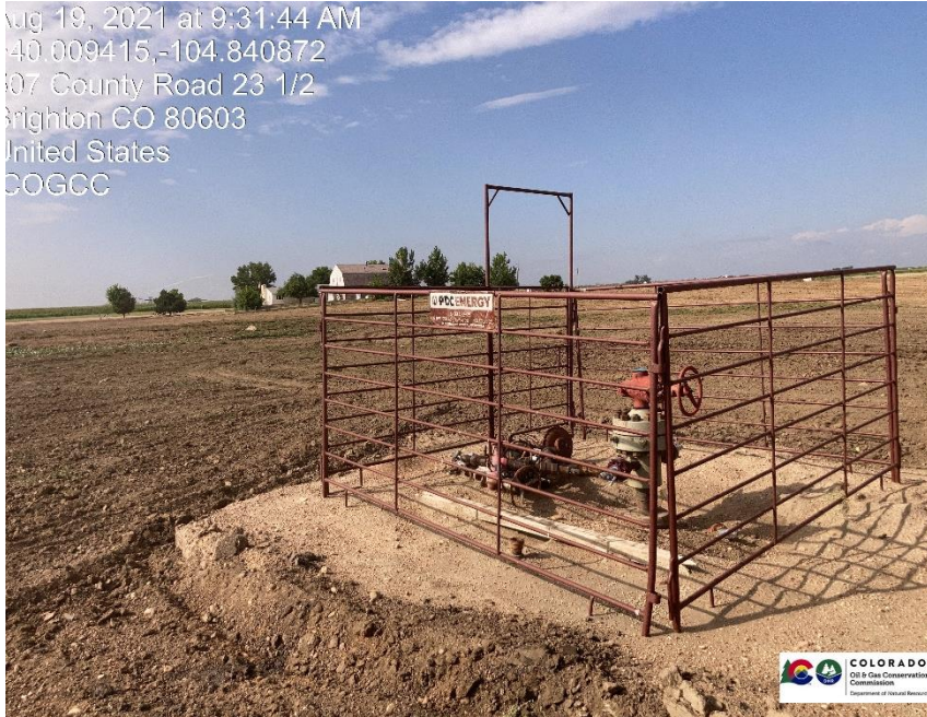
Pic 3 Wellhead is TA, production equipment is laying next to wellhead.
