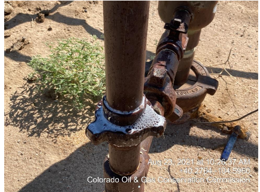
Photo #4 Leaking union & Weeds
