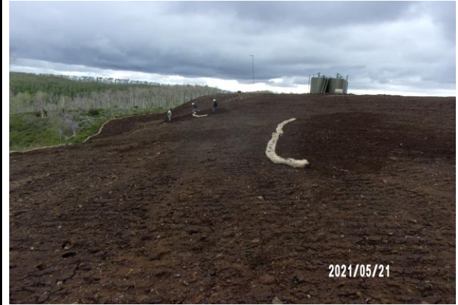
Wattle Installed below Minor Erosion
