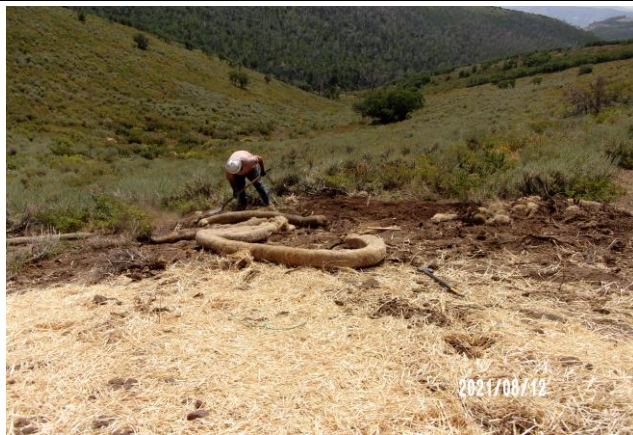
Replacing Section of Wattle on the CC 610-22-43 Pad
