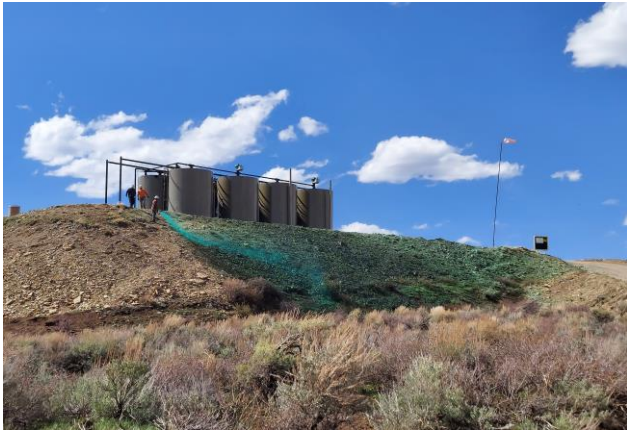
Applying Hydroseed Mix over Cut Slope
