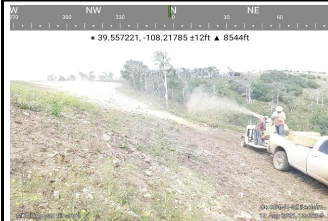
Applying Straw Mulch to the CC 604-41-32 Pad
