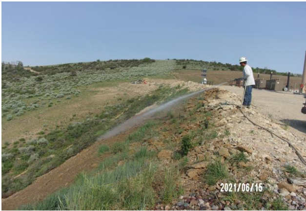
Applying Additional Water, Nutrients, and Soil Amenities on CC 604-41-32 Fill Slope
