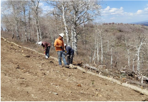
Maintaining Perimeter Wattle on CC 604-41-32
