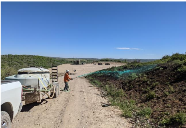
Irrigating the CC 697-03-07 Access Road Cut Slope
