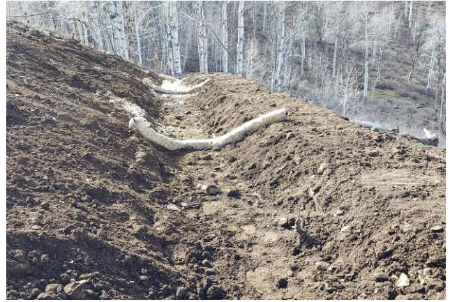
New Sediment Trap Outlet Installed
