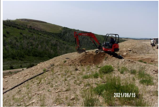
Installing Flex Hose Outlet on CC 604-12-13 Annex Pad
