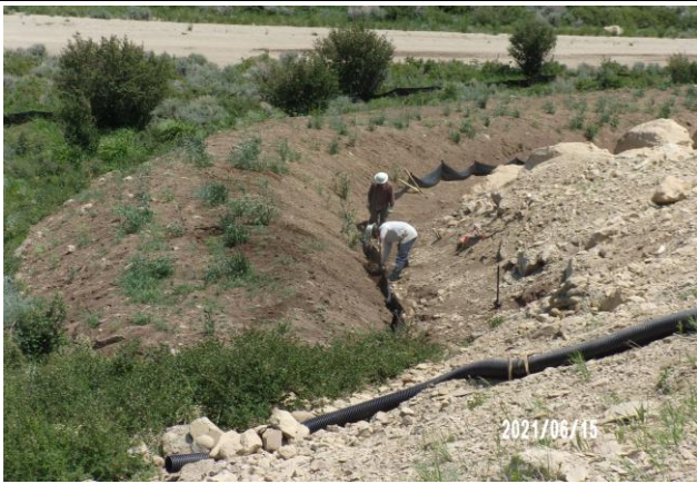
Mending Silt Fence Installed on CC 604-12-13 Annex Pad
