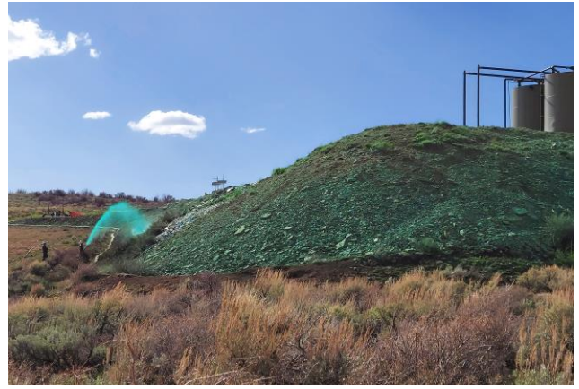
Applying Hydroseed Mix over Cut Slope
