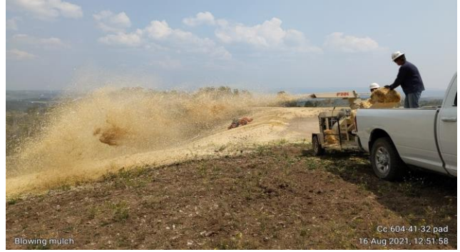
Blowing Straw Mulch on CC 604-41-32 Pad
