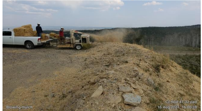
Blowing Straw Mulch on CC 604-41-32 Pad
