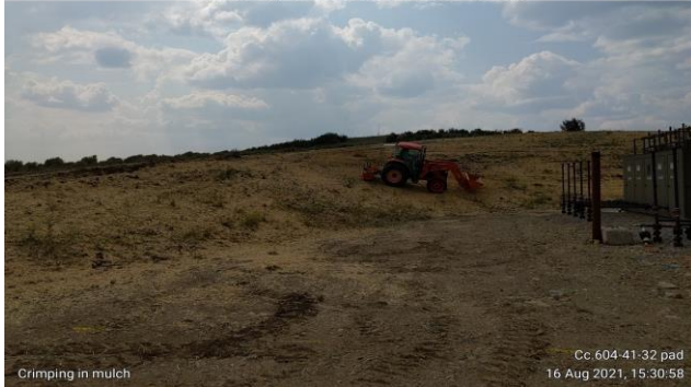
Crimping Straw Mulch on CC 604-41-32 Pad
