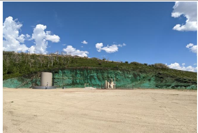
Location after Treating Cut Slope with Liquid Amenities and Nutrients
