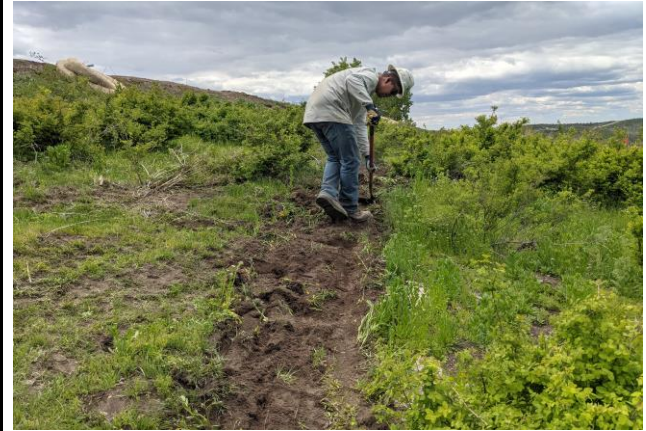
Installing Trench for Wattle Installation by Hand
