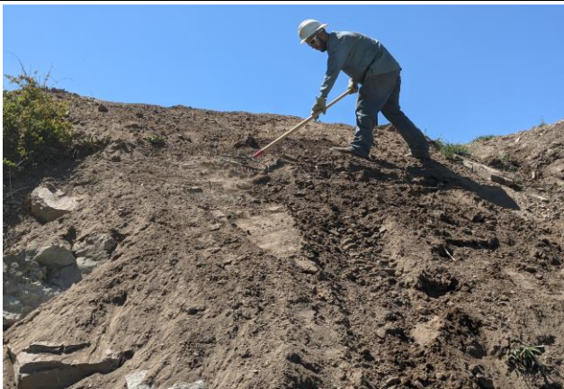
Hand Raking Seed to Incorporate into Soil
