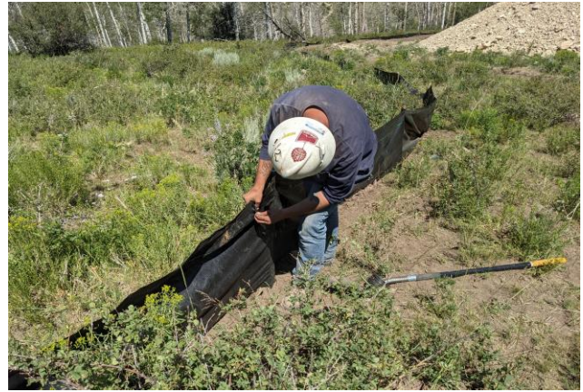
Repairing Silt Fence on CC 697-03-07 Pad
