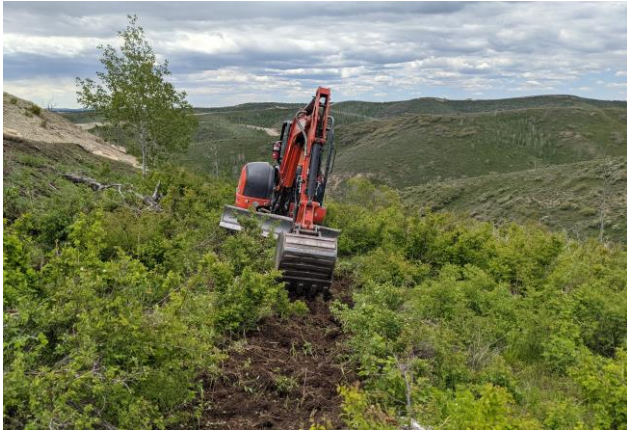
Clearing Vegetation in Preparation for Wattle Installation
