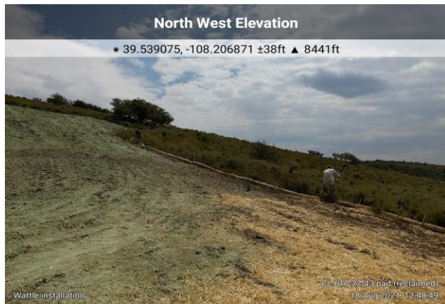
Installing Excelsior Wattle around the Perimeter of the Reclaimed CC 610-22-43 Location
