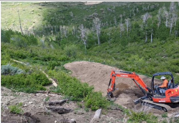
Maintaining Sediment Trap near the Pad Entrance
