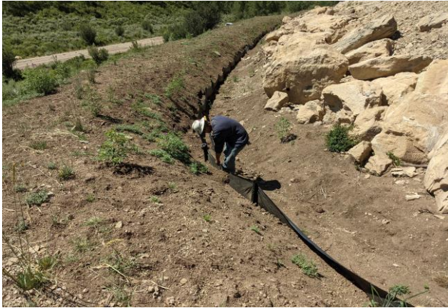
Mending Silt Fence on CC 604-12-13 Annex Pad
