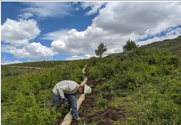
Stringing Out Wattle to be Installed
