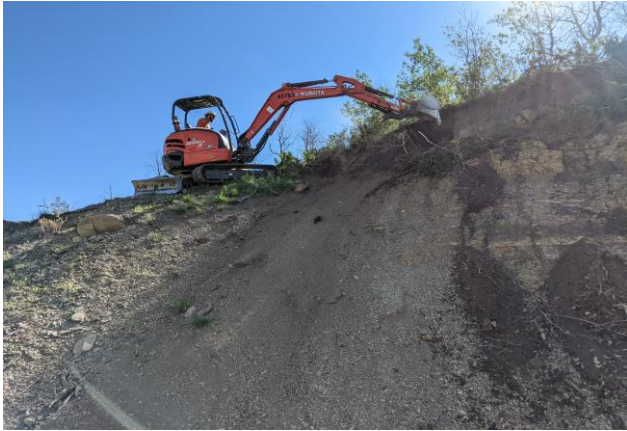
Shaping Verticle Cut above Cut Slope
