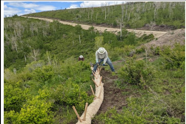
Installing Wattle on the CC 610-22-43 Pad
