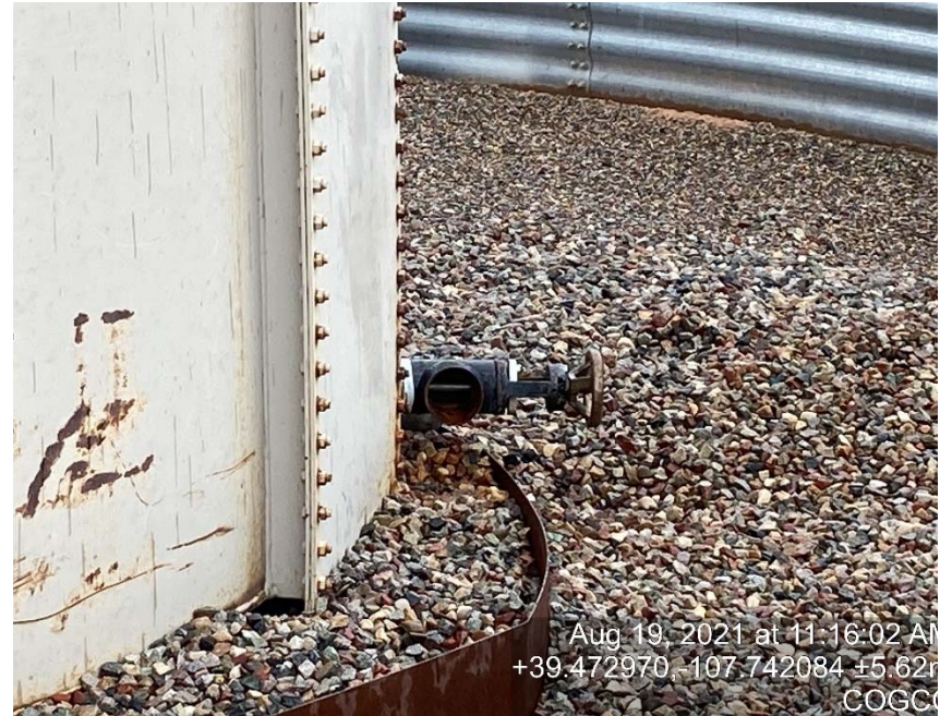
Load out line missing cap/bull plug
