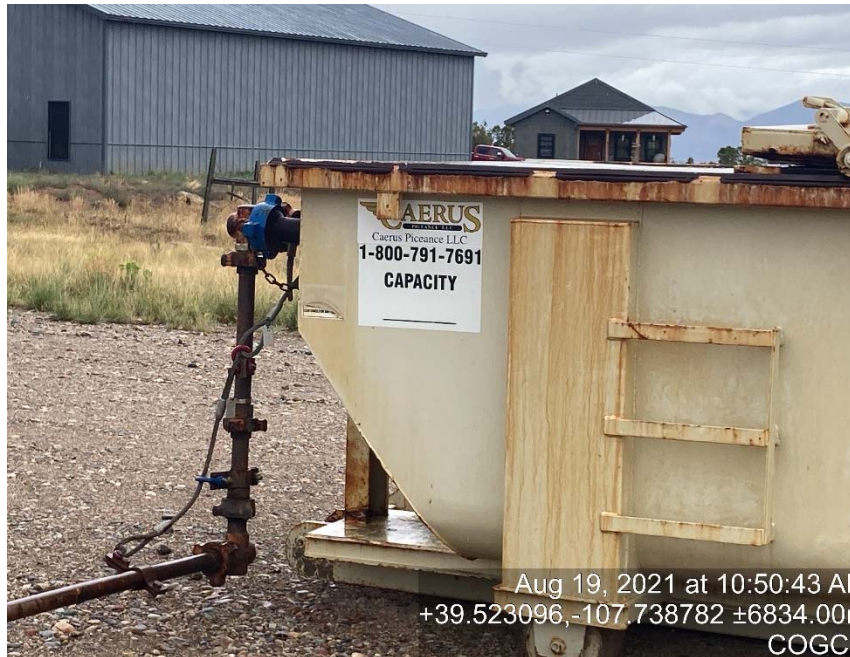
Roll top tank missing signage
