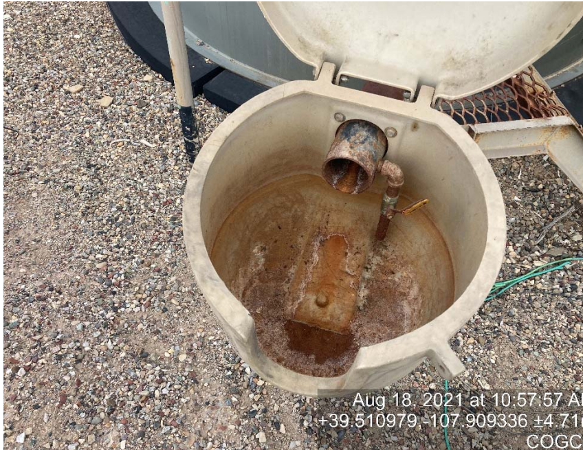
Load out line missing bull plug/cap
