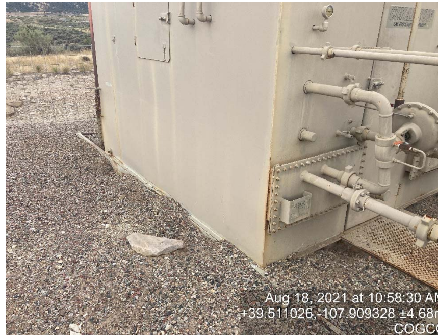
Separator bath missing labeling
