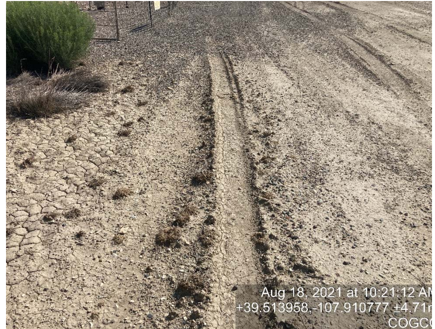
Lack of stabilization/compaction
