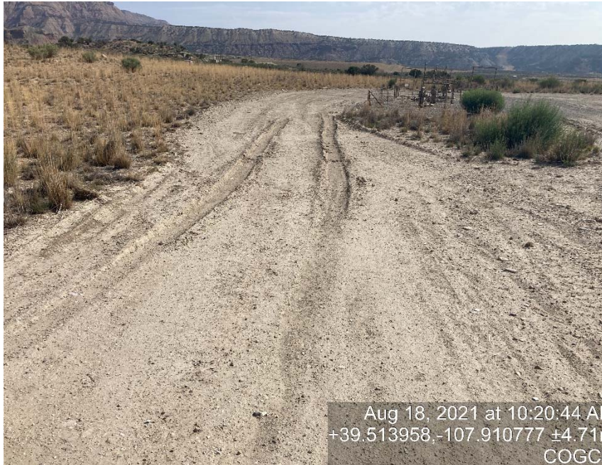
Lack of stabilization/compaction
