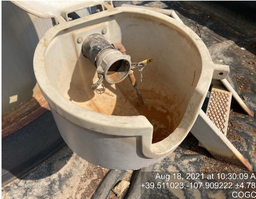
Load out lines missing bull plugs/caps
