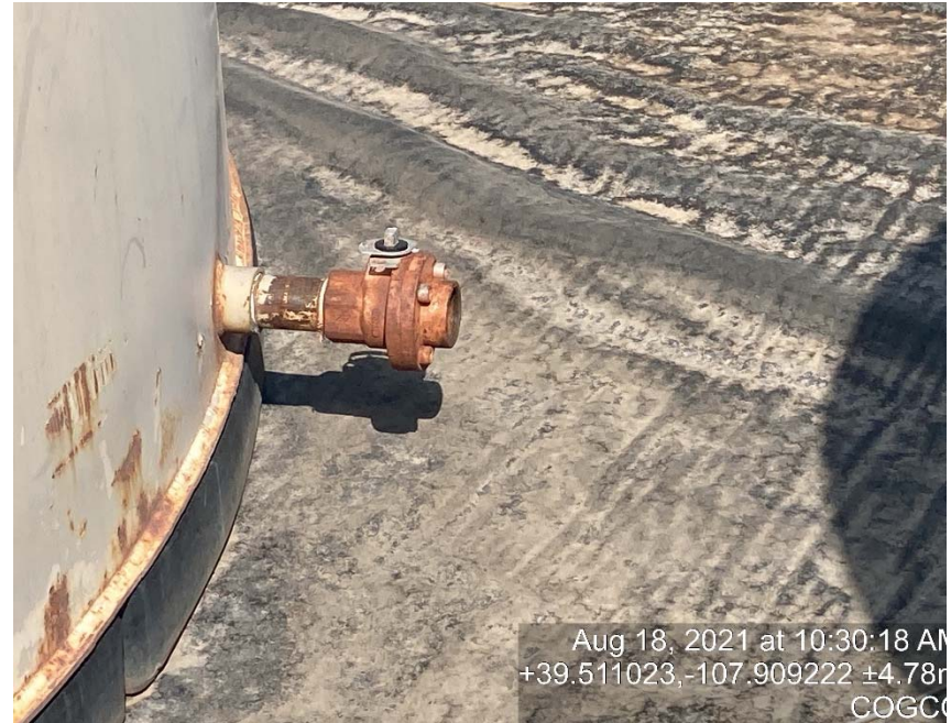
Load out lines missing bull plugs/caps
