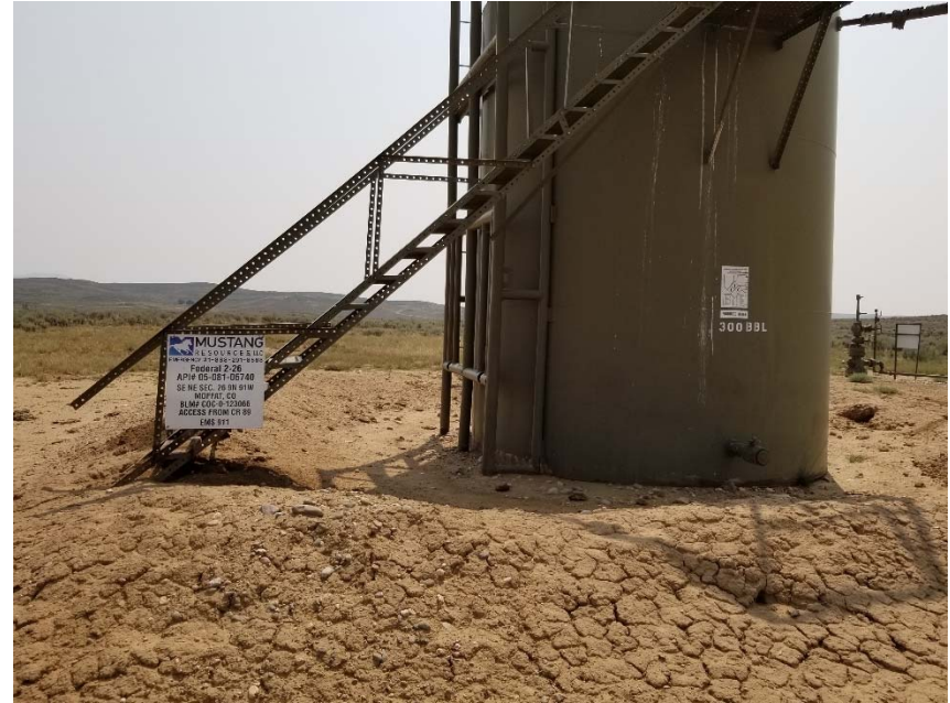
Photo 2. Signs not updated to current operator. Incomplete tank label. Animal burrows in berms.
