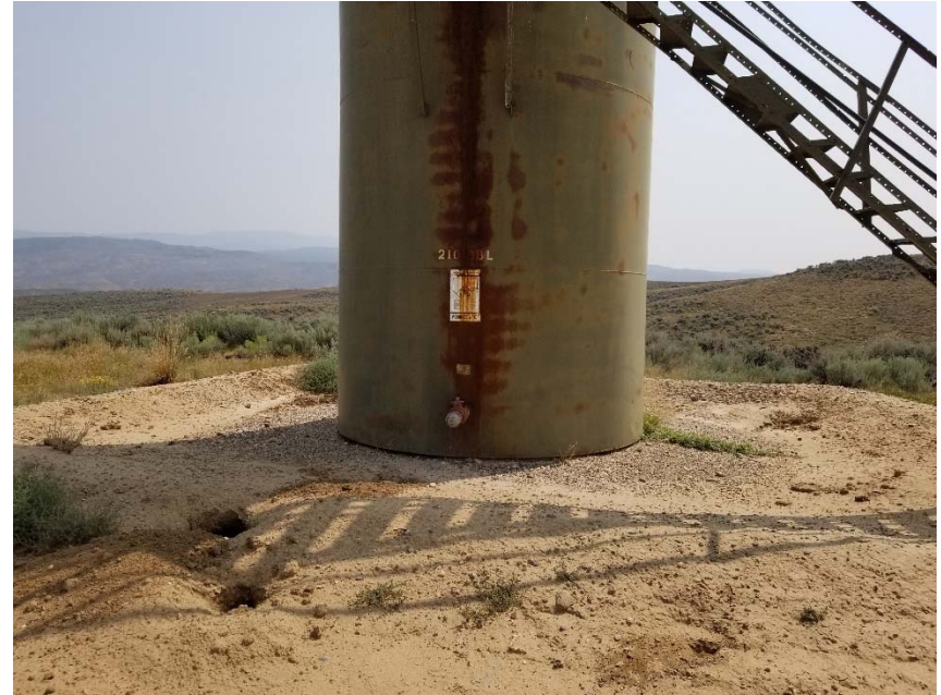
Photo 3. Tank label faded. Animal burrows in berm.
