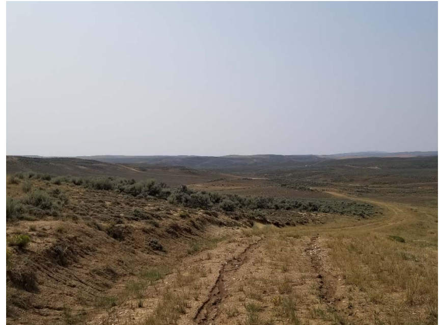
Photo 3. Sediment migration on overgrown access road.
