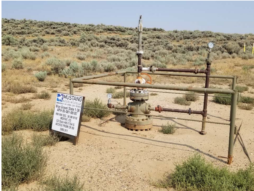
Photo 2. Signs still have previous operator information. No bradenhead access apparent. Annual weeds.
