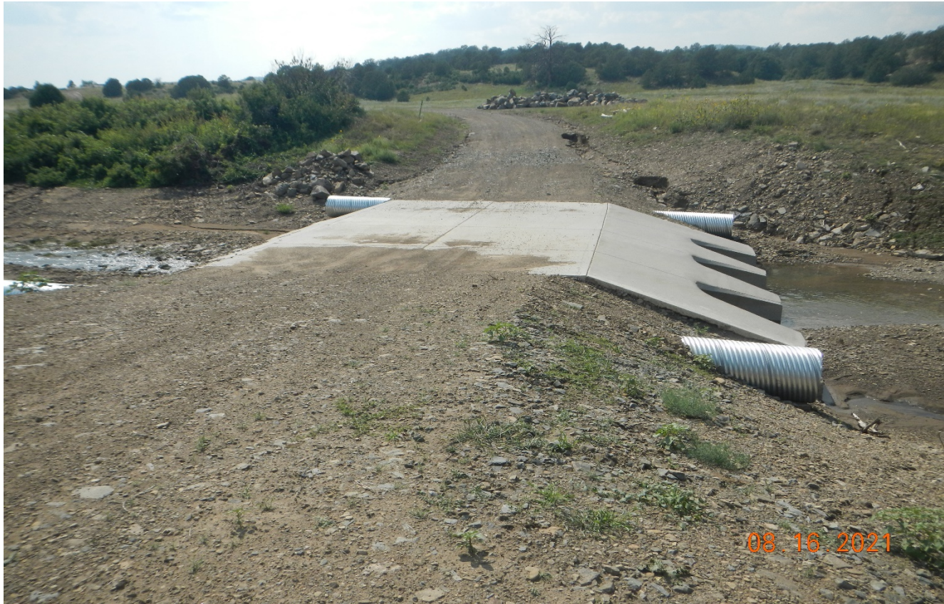
Photo 2. Facing back west at the stream crossing. There are two additional culverts installed.
