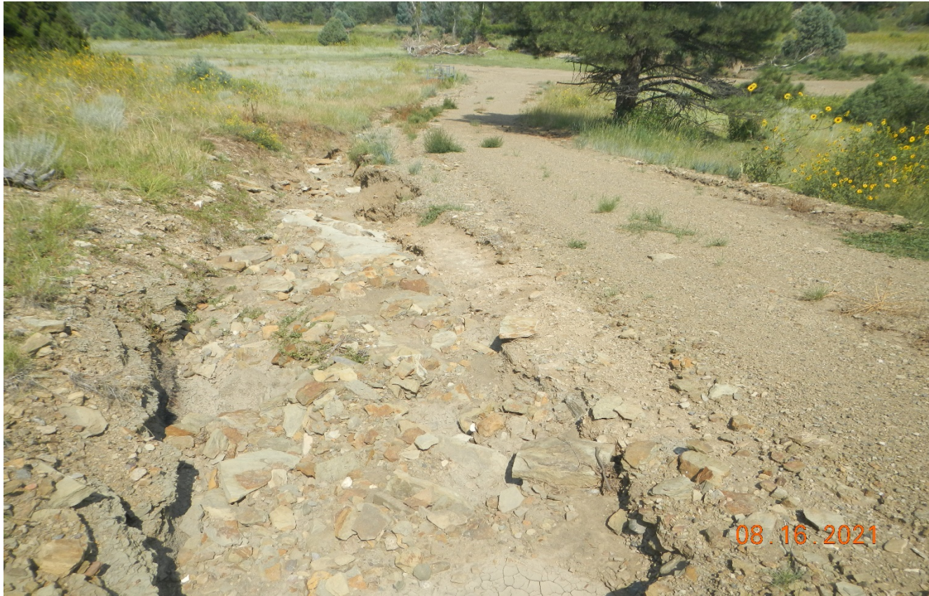
Photo 4. Facing back down the road. The erosion along the road side will need to be repaired and stabilized.
