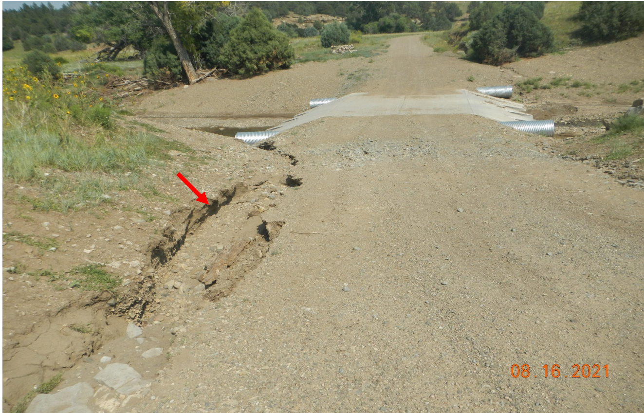
Photo 1. Facing east toward the access road stream crossing which was washed out during the flood event. The road side area shown at red arrow is beginning to erode and needs to be stabilized.
