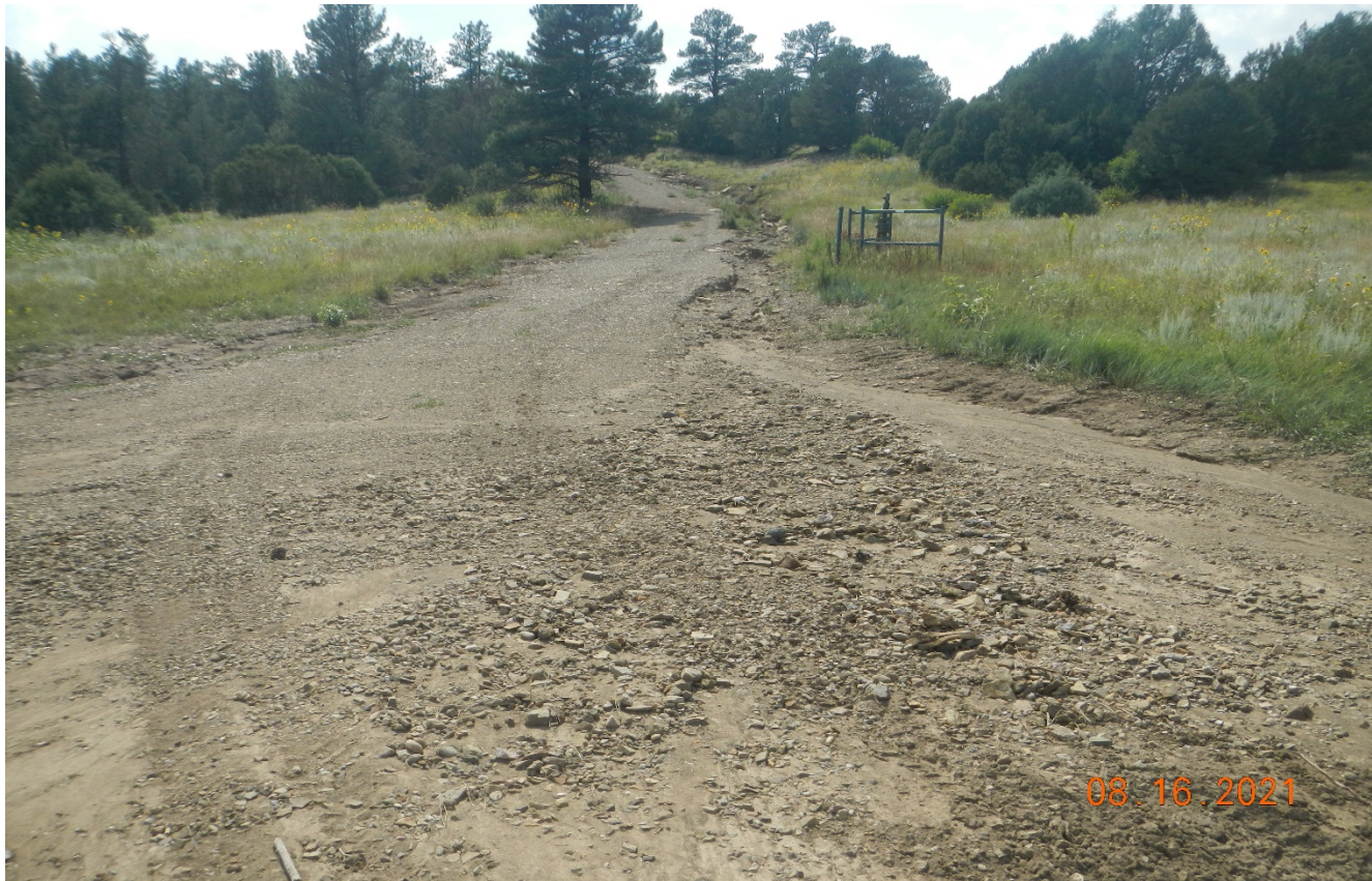
Photo 3. Facing southwest toward the access road. Stormwater further up the road is directed toward this area. There are insufficient BMP's along the road side.
