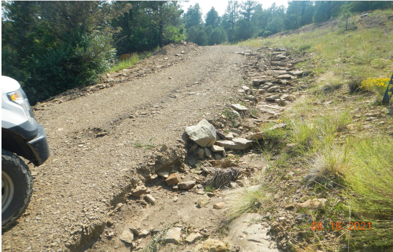
Photo 5. Further up the access road. The erosion along the road side will need to be repaired and stabilized.
