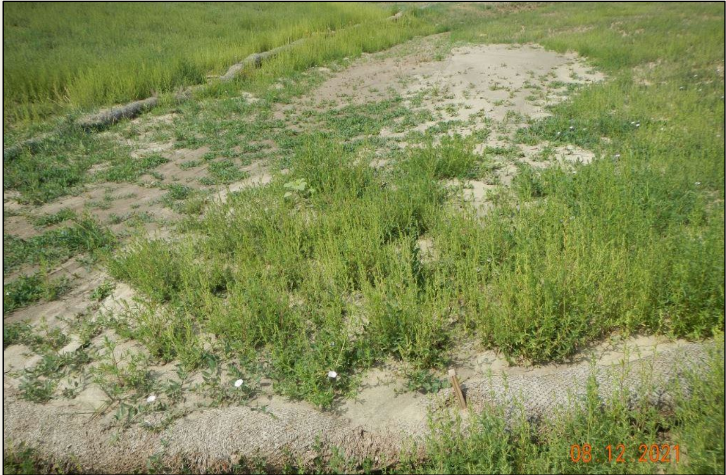
Photo 4. View of straw wattles filled with sediment needing replacement and maintenance.
