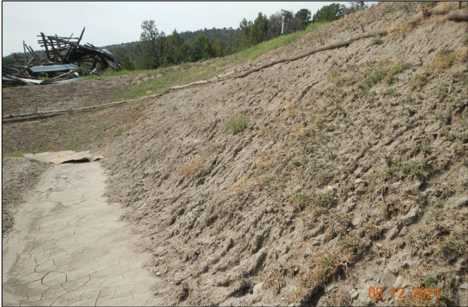
Photo 5. View of area along the well pad cut-slope with rilling and debris deposition, facing southward.
