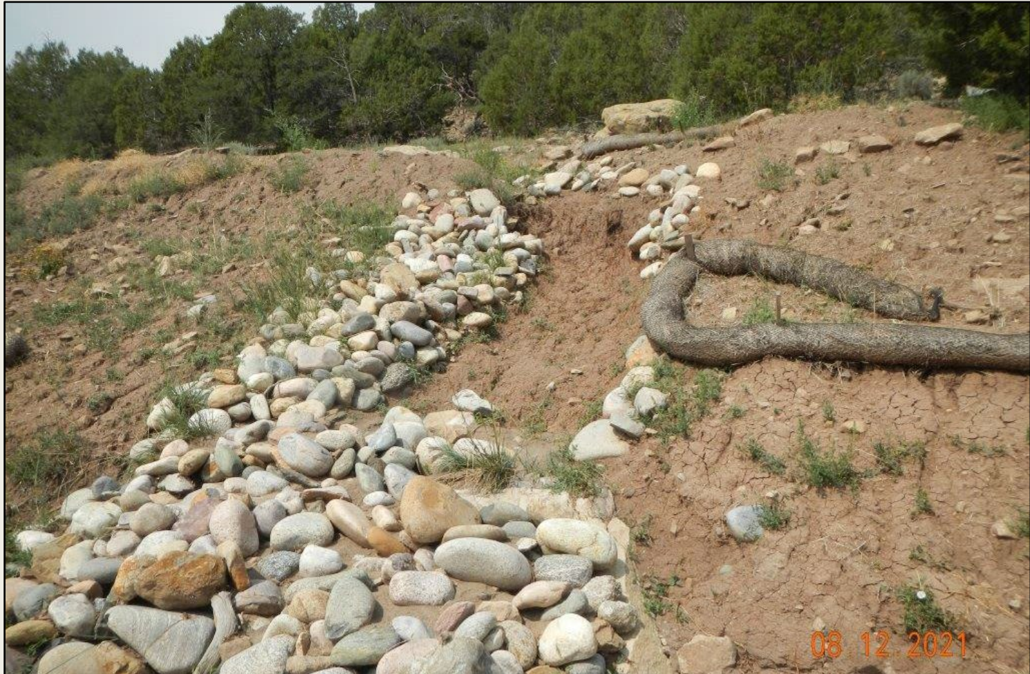
Photo 8. View of eroded BMP within the northwestern project area where cobble and wattles are washed out.
