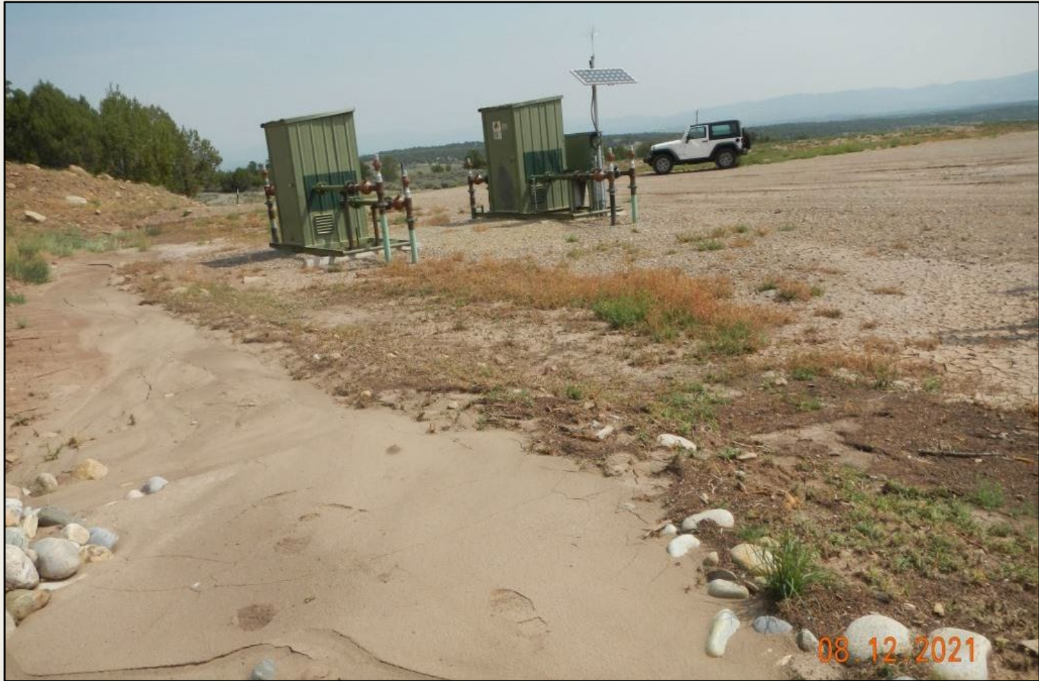
Photo 9. View of sediment deposition observed below failed BMP in Photo 8.
