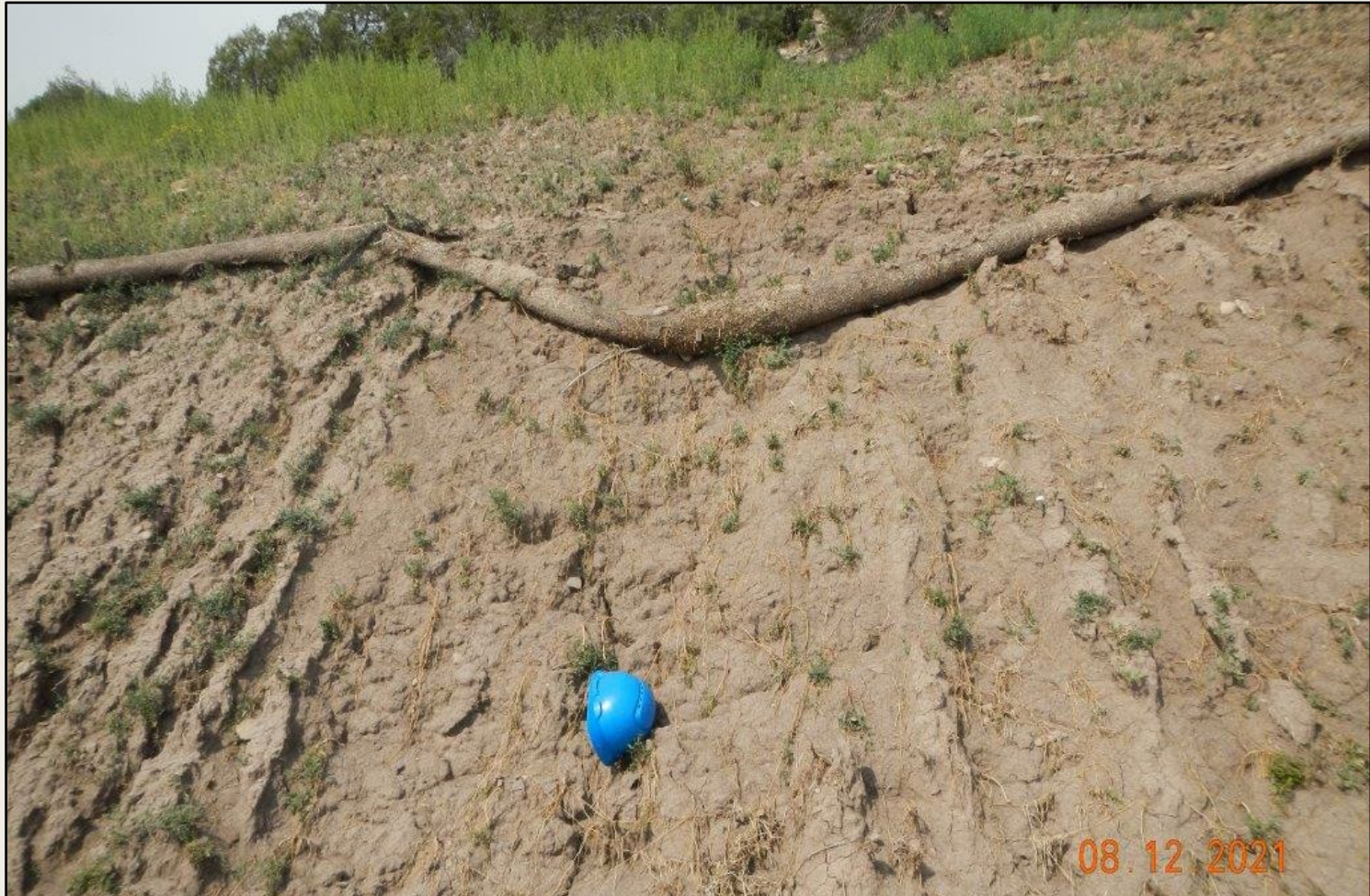
Photo 6. Another view of area on the well pad cut-slope with significant rilling and channeling (up to 1 foot wide and deep).
