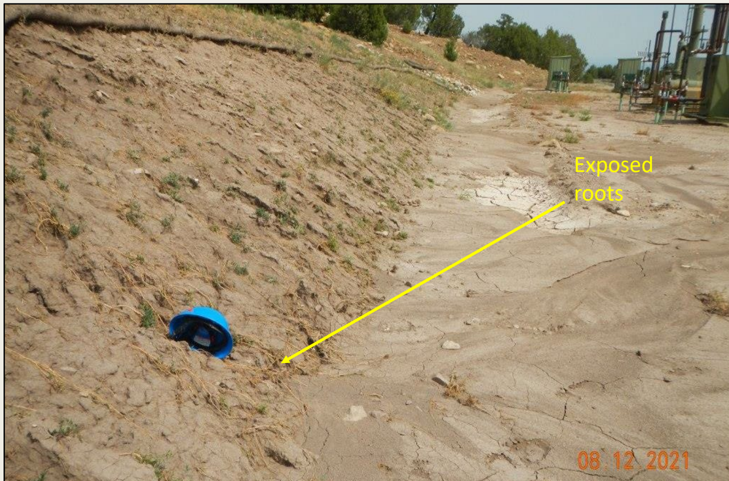
Photo 7. View of rilling, exposed roots, and sediment deposition at the toe of the cut-slope.
