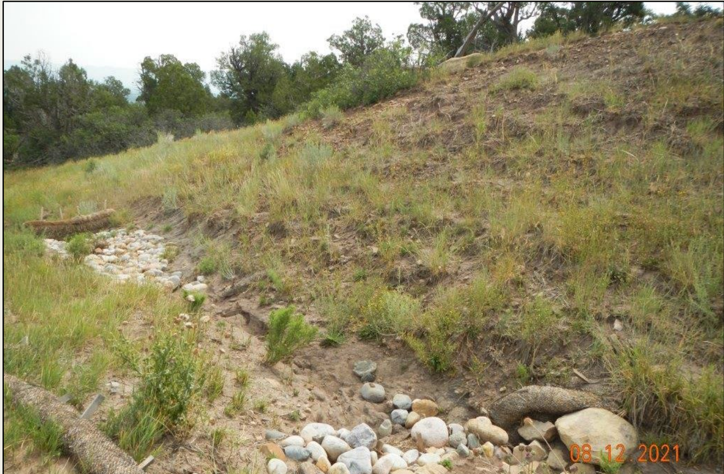
Photo 4. View of stormwater BMPs within the southeastern project area straw bales and wattles need maintenance and reinforcement.
