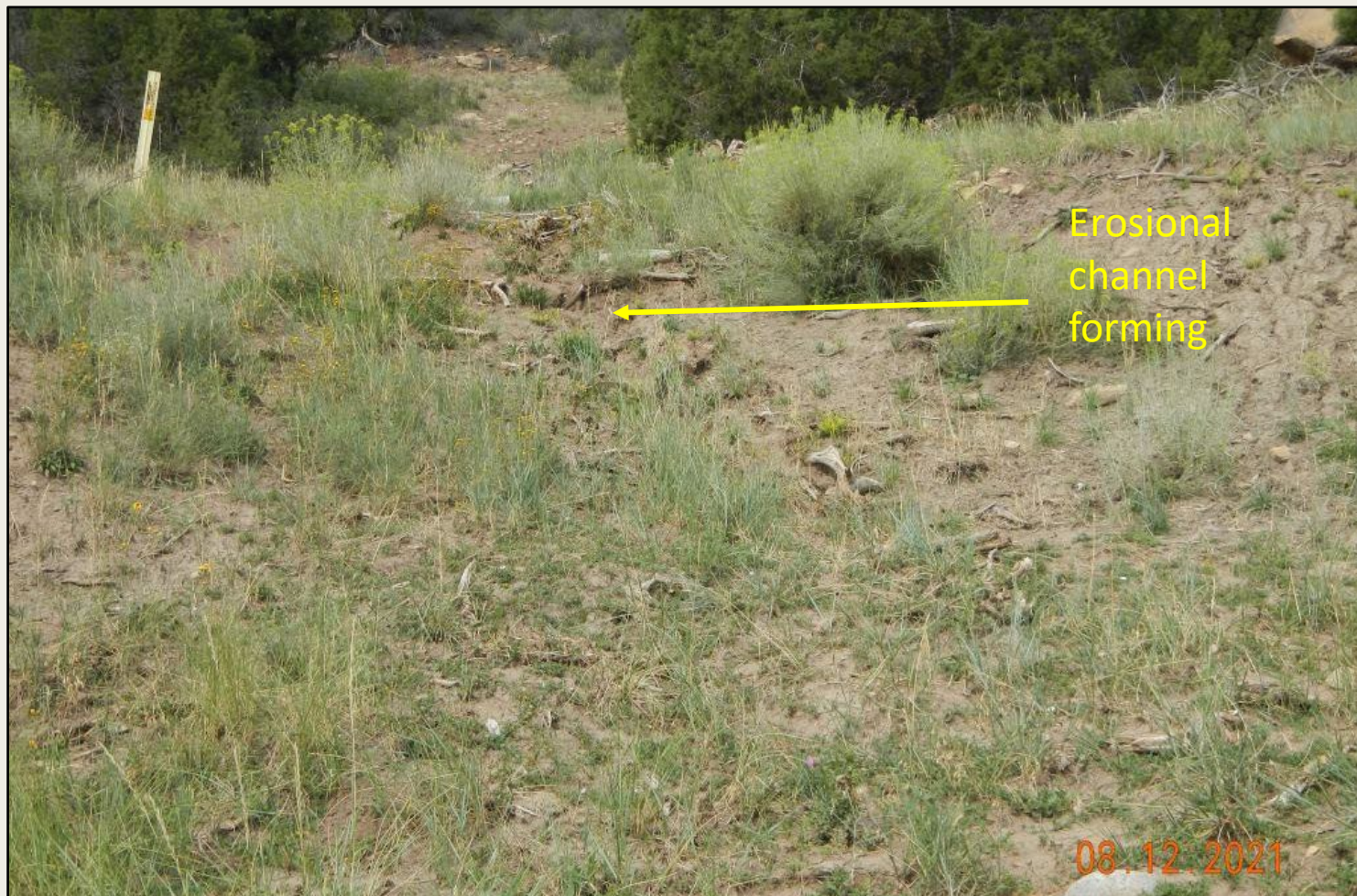
Photo 3. View of erosional channel forming within the flowline ROW, approximately 1 foot wide and deep, needs stabilization.
