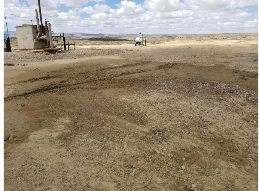
Photo 6. Sediment transported onto location. Close up of photo 5.
