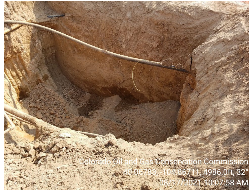
Photo 2 – Spill excavation is open. Impacts remain in-situ. Seepage of groundwater was observed in the lowest point on the floor/sidewall of the excavation.
