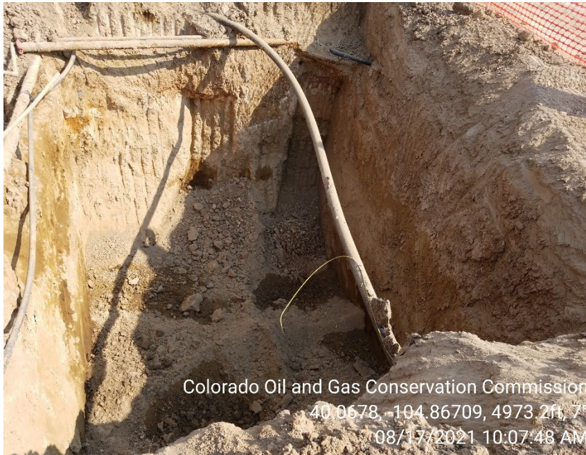
Photo 1 – Spill excavation is open. Impacts remain in-situ.
