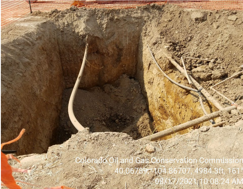
Photo 3 – Spill excavation is open. Impacts remain in-situ.
