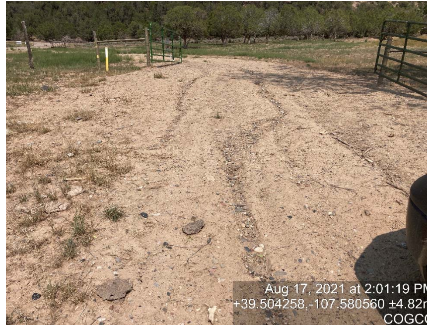
Lack of stabilization/compaction/erosion
