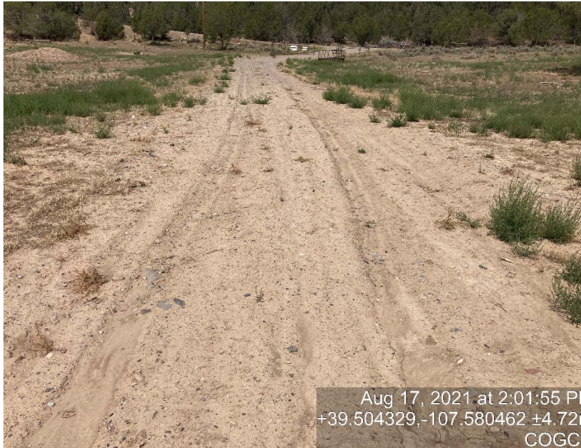
Lack of stabilization/compaction/erosion
