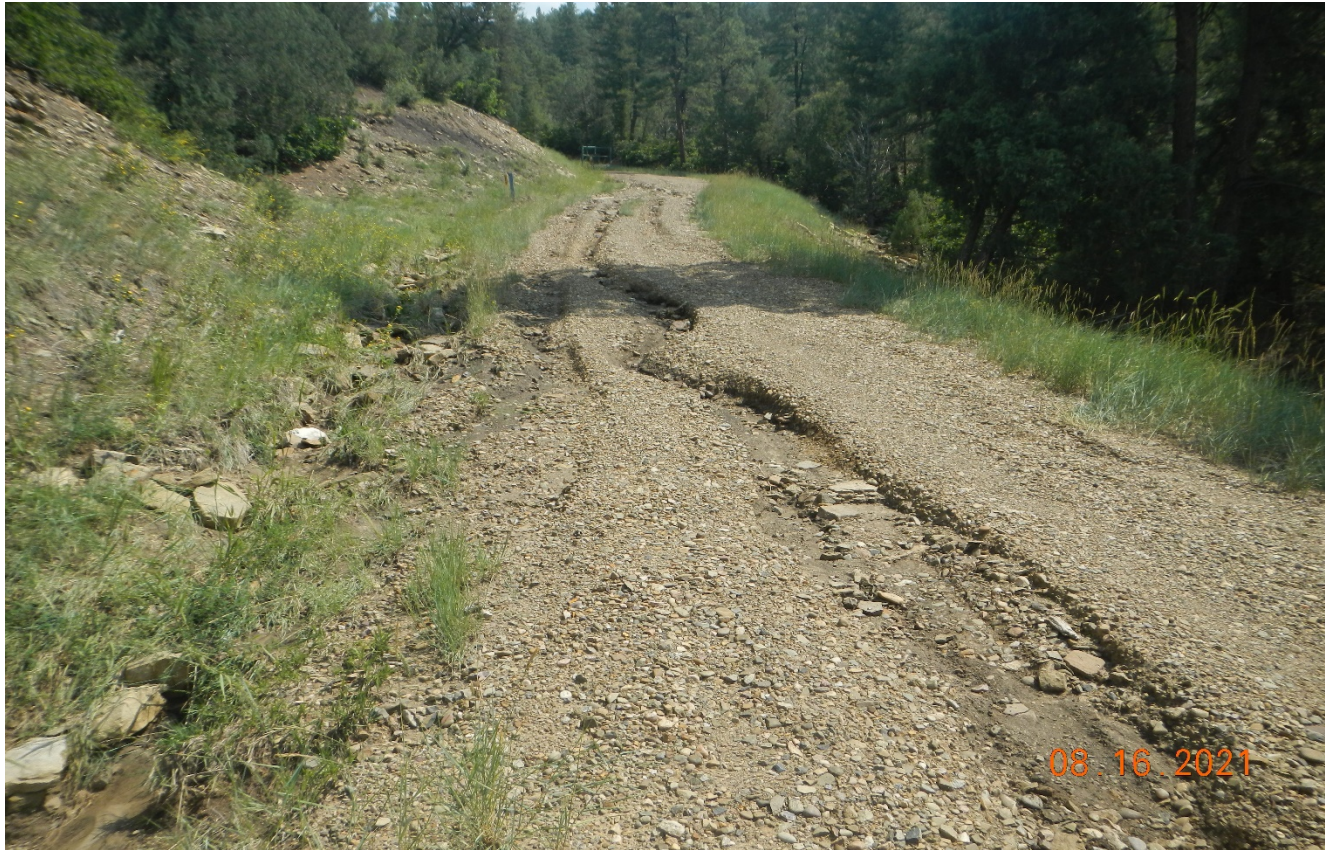
Photo 1. There is stormwater erosion occurring down the road. The road needs to be repaired and stormwater diverted off the road and toward culverts.
