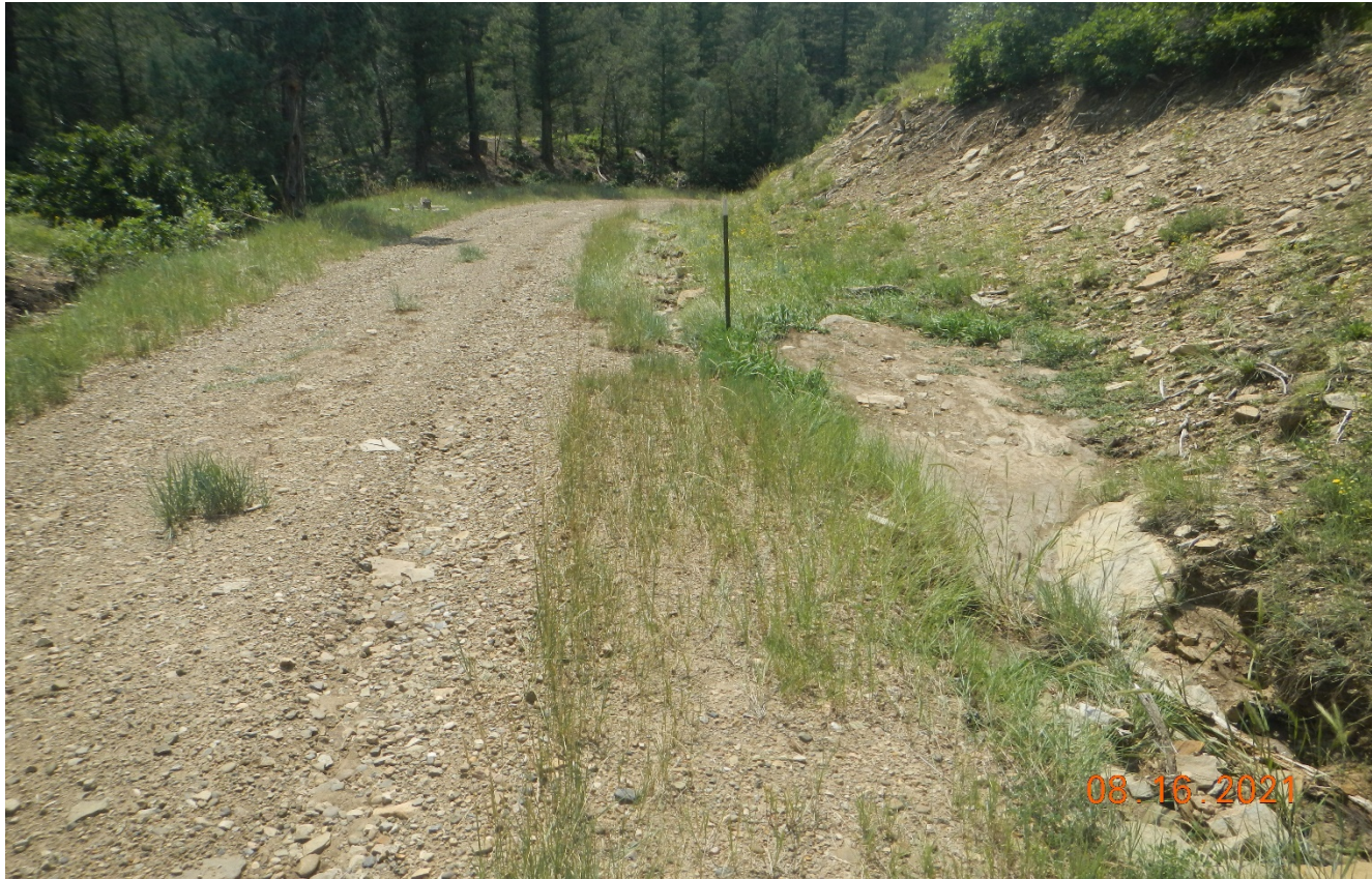
Photo 2. There are culverts along the road that have filled in with sediment and need maintenance.
