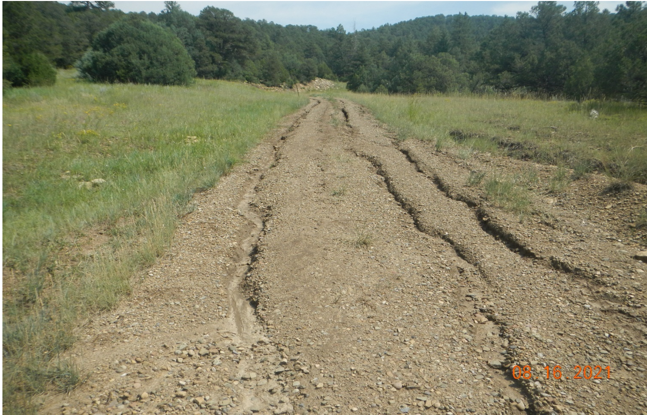
Photo 3. There is stormwater erosion occurring down the road. The road needs to be repaired and stormwater diverted off the road.
