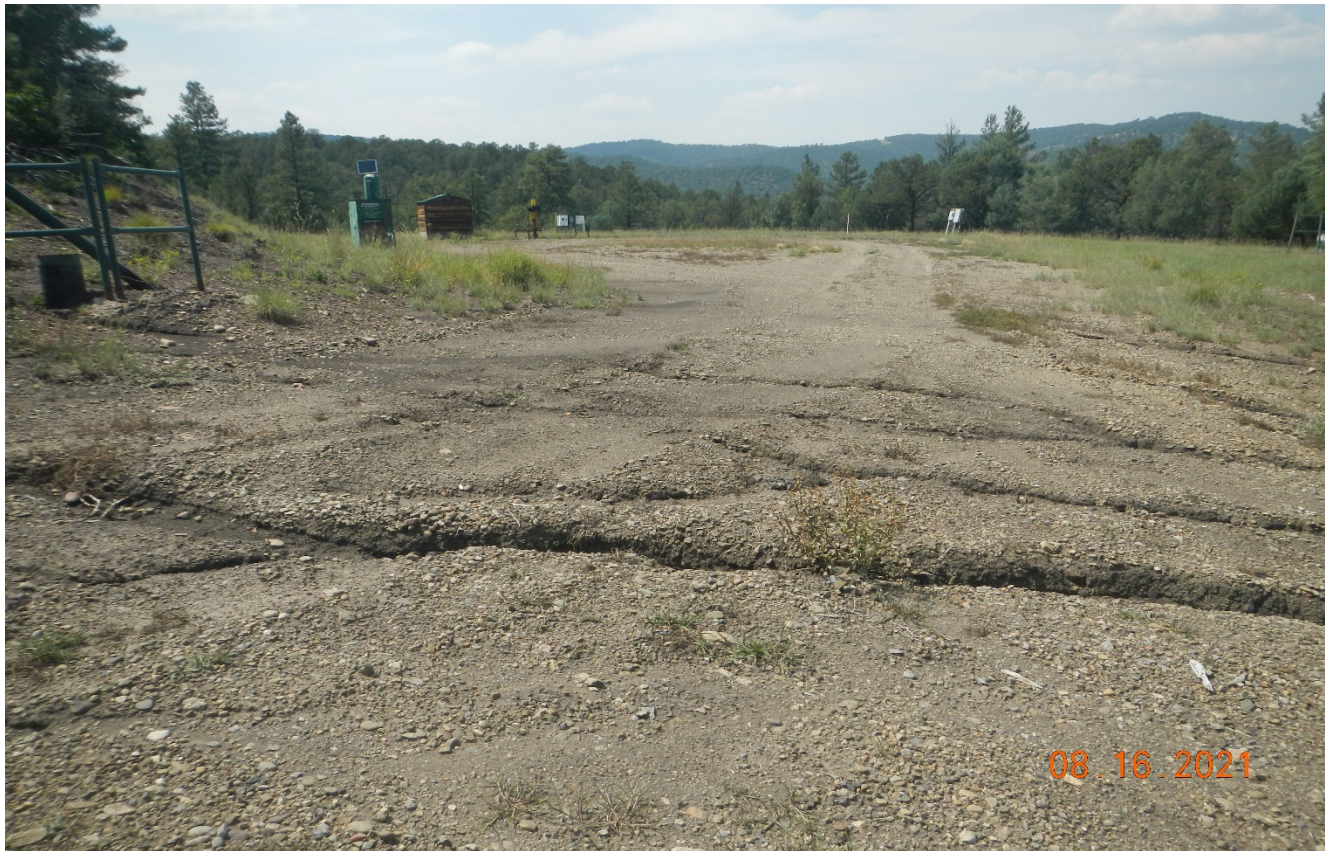
Photo 4. Facing west toward the well site. There is erosion across the access road which needs to be repaired.
