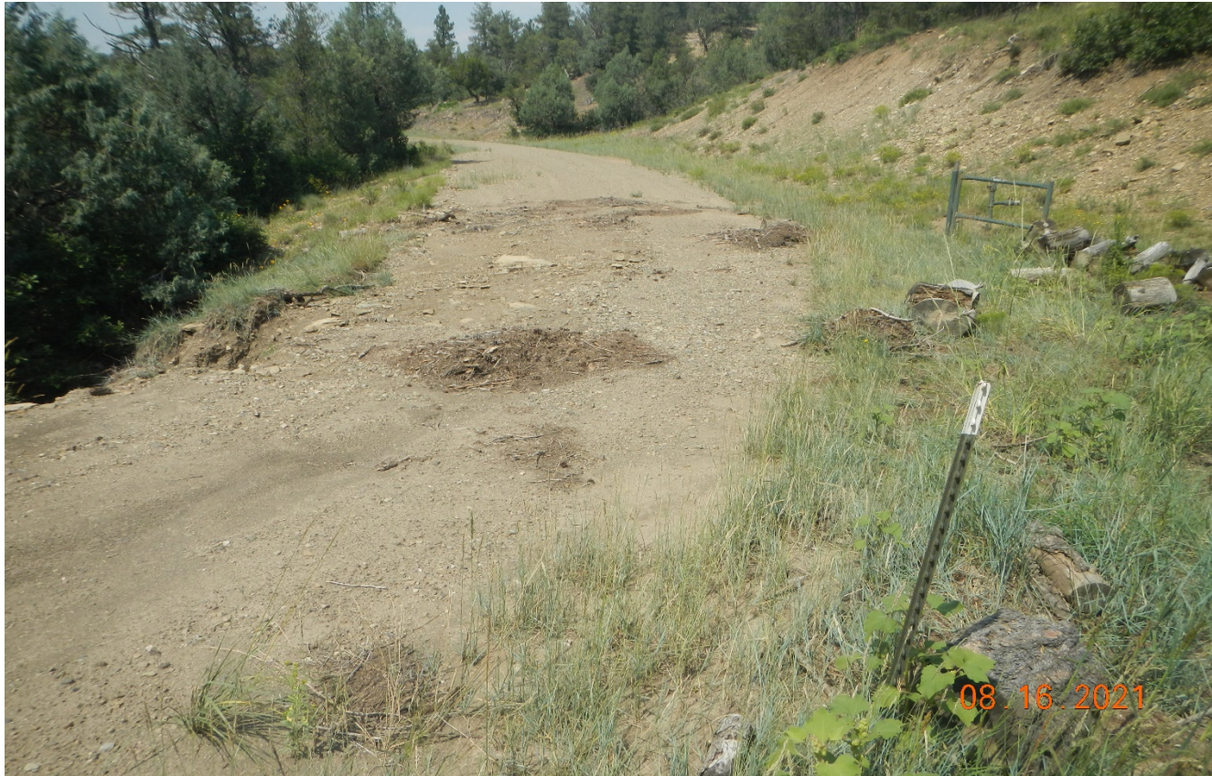
Photo 2. Further along the road at this drainage, the culvert plugged up and stormwater had flown over the road. The culvert needs to be repaired at this drainage area.
