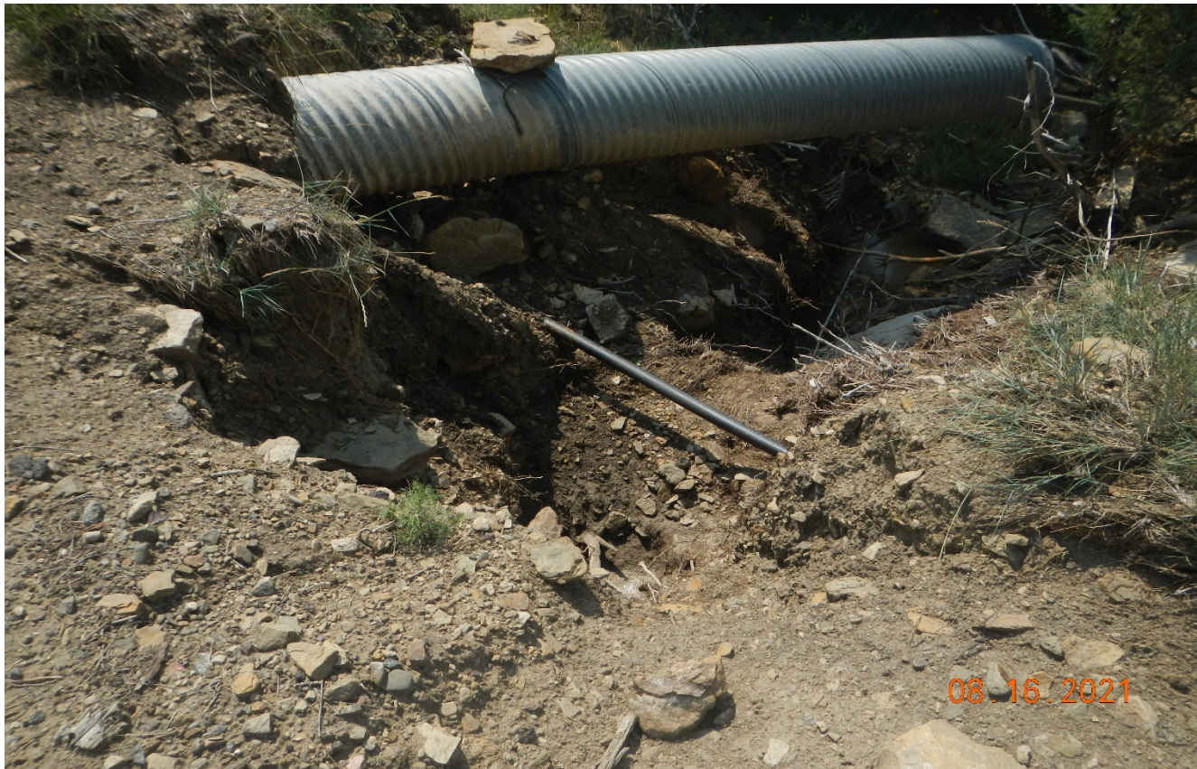
Photo 3. The same culvert outlet has eroded and exposed a pipeline. This area needs to be repaired.
