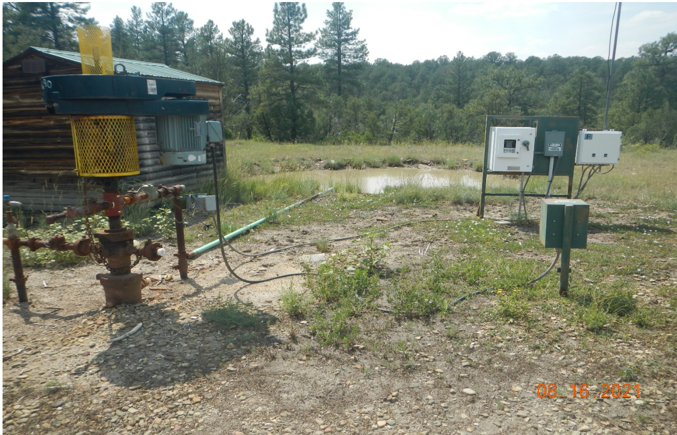
Photo 5. Facing toward the well and PW pit. The water level is near 2 ft. freeboard.
