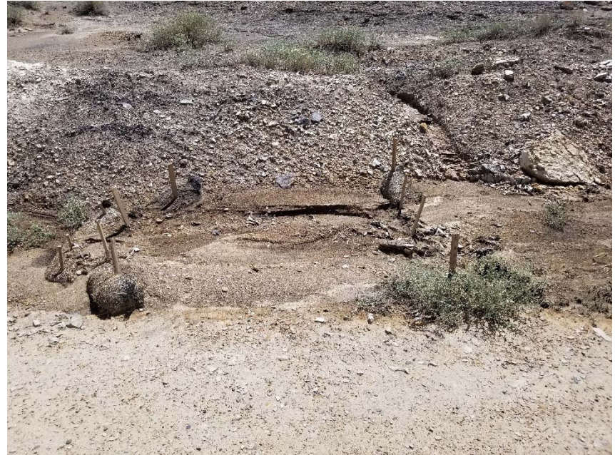
Photo 3. Failed BMPs in ditch along access road.
