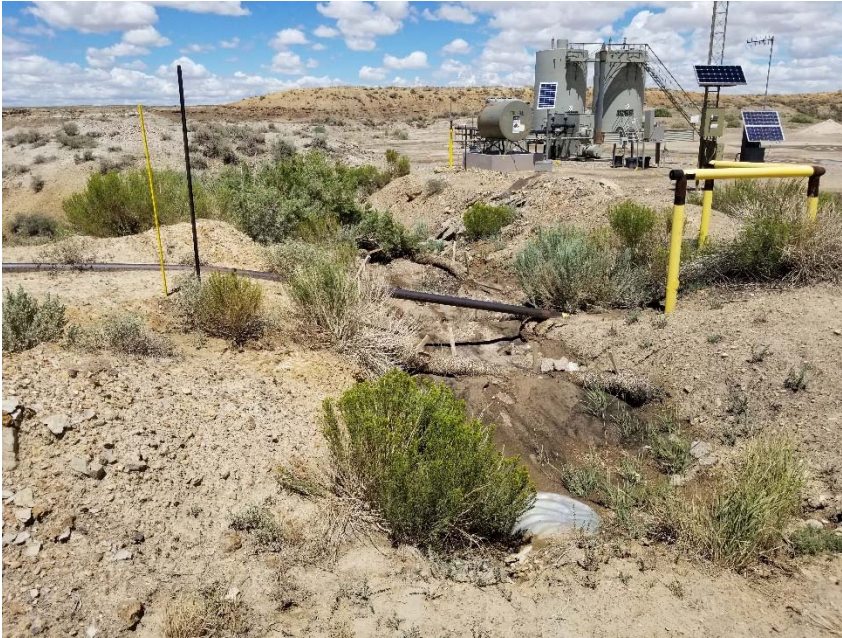
Photo 2. Failed BMPs at location entrance.
