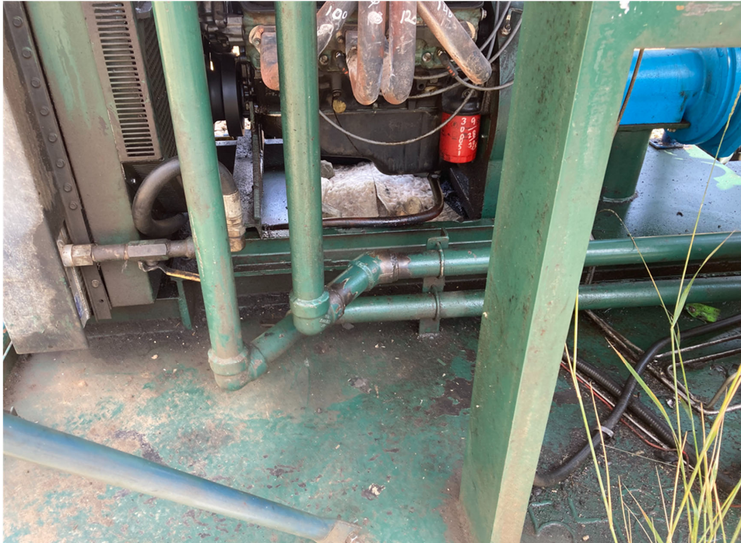
PHOTO 3: THE LEAK ON THE COMPRESSOR WAS REPAIRED. ALL FITTINGS ARE SECURLY FASTENED. THE FLUID ACCUMULATION WAS REMOVED FROM THE CONTAINMENT.
