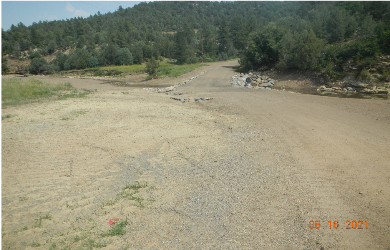
Photo 1. Facing east toward the access road stream crossing which was washed out during the flood event.
