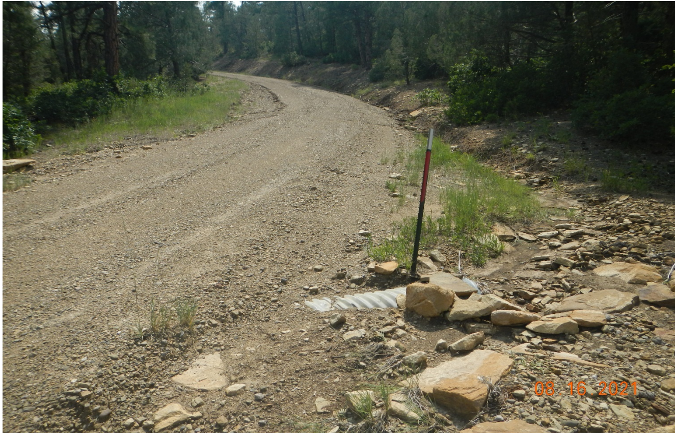
Photo 7. Another culvert further along the road is filled in with sediment.
