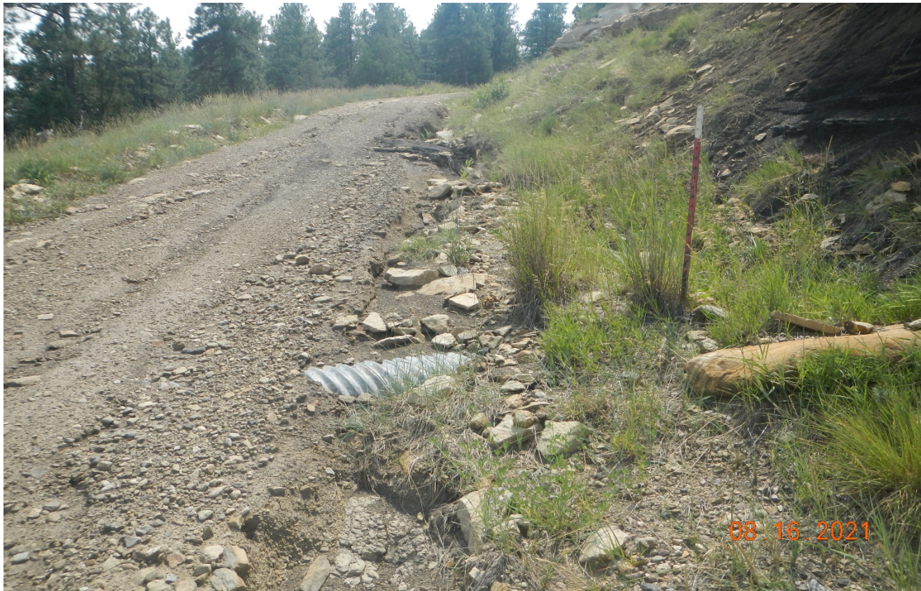
Photo 5. The culverts along the access road are filled in with sediment.
