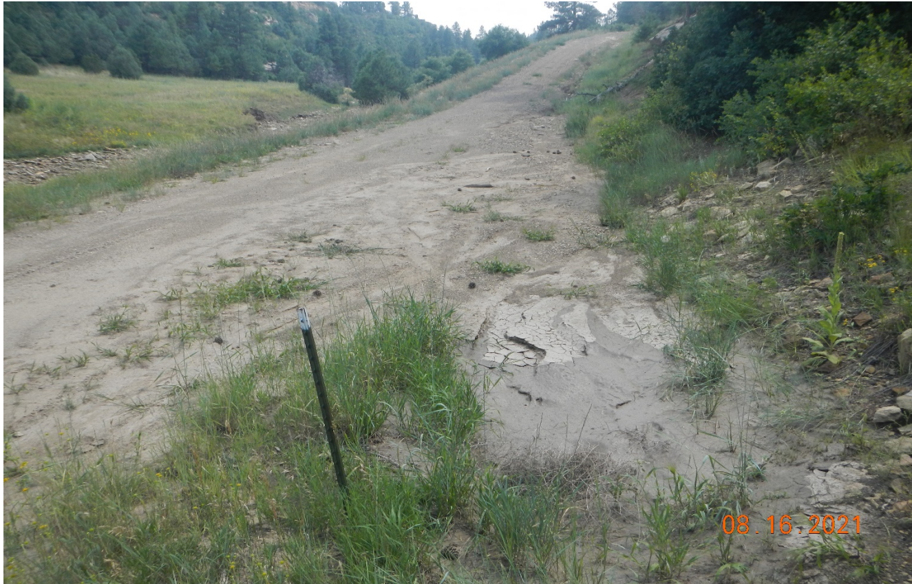
Photo 4. Facing southeast along the access road. The culverts along the access road are filled in with sediment.
