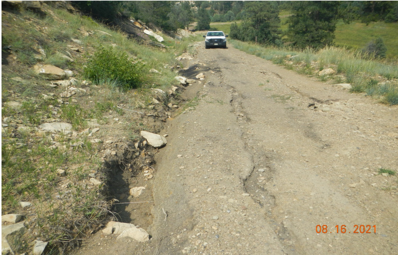
Photo 6. Facing back down the road. There is erosion along the road side and stormwater is bypassing culverts which will cause further erosion. BMP's need to be repaired.
