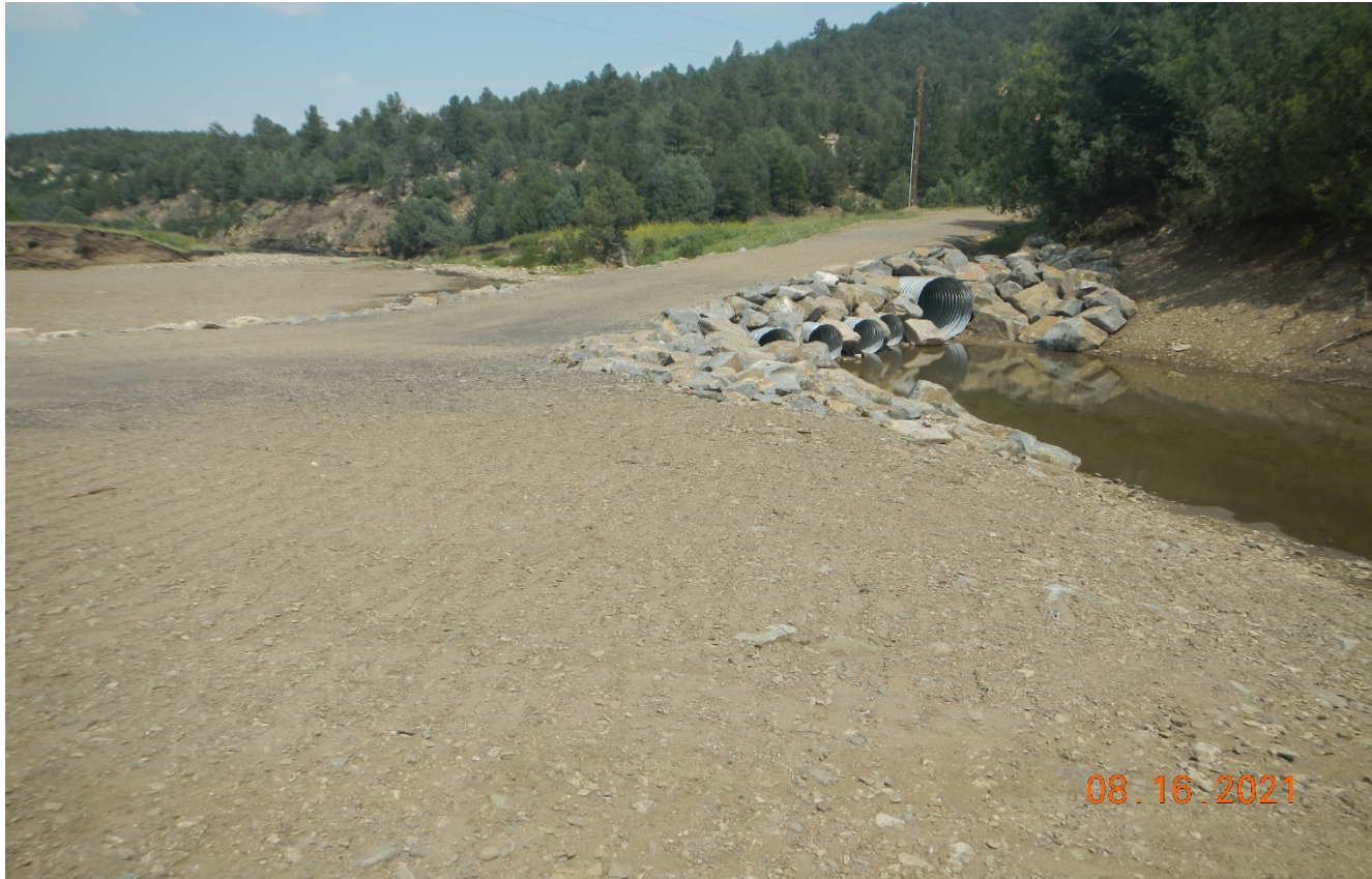
Photo 2. There are multiple culverts installed and rock rip/rap was installed for bank stabilization. The culverts are multiple sizes and it is unknown if this was an adequate engineered practice.
