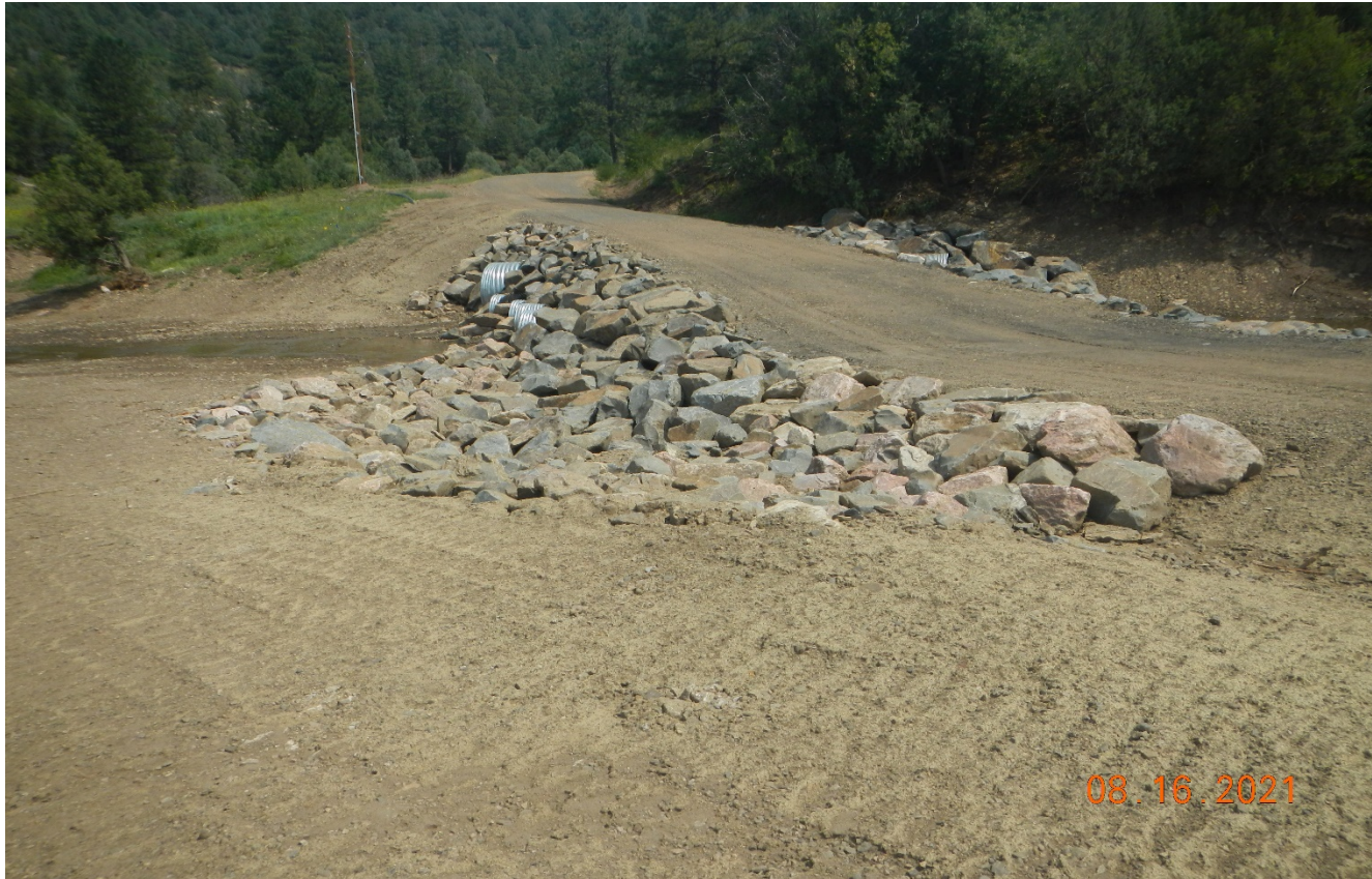
Photo 3. Facing east at the stream crossing. There is bank stabilization along the outlet side of the stream crossing.
