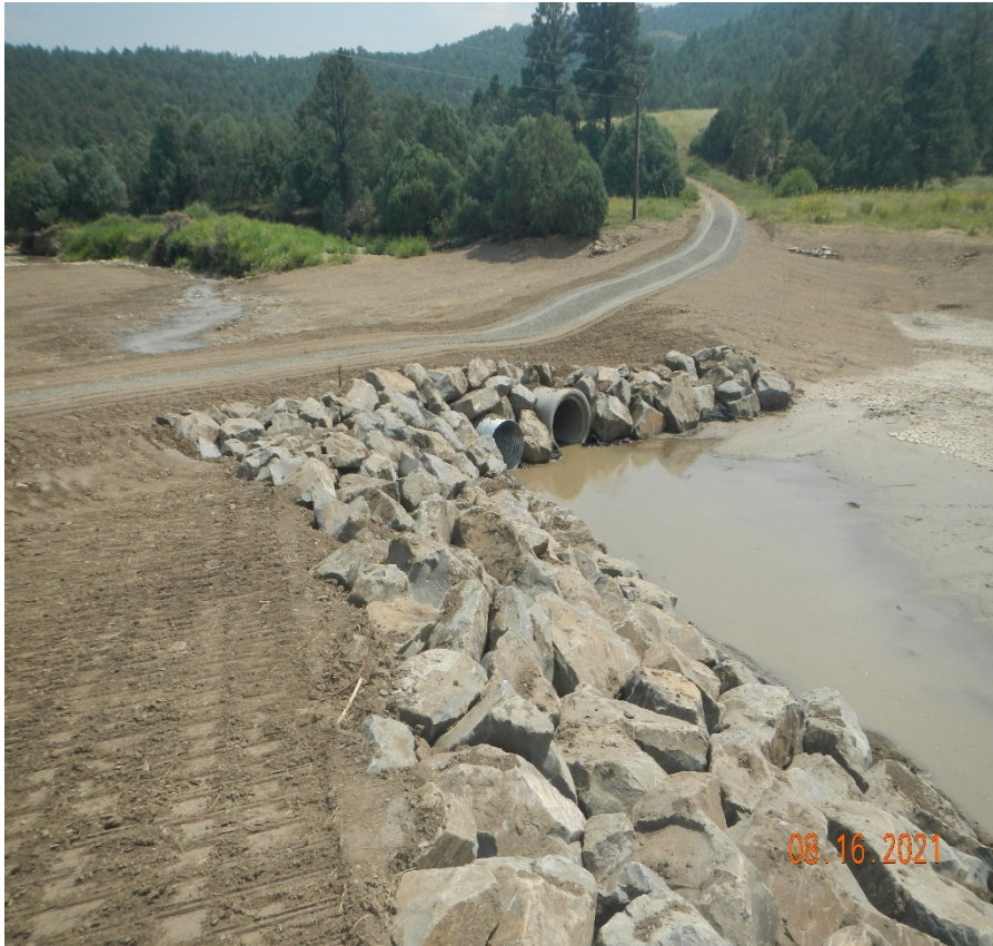
Photo 2. There are two culverts installed at the stream crossing. This appears to be inadequate as the prior cement culvert shown in the photo on the right had 3 large outlets.
