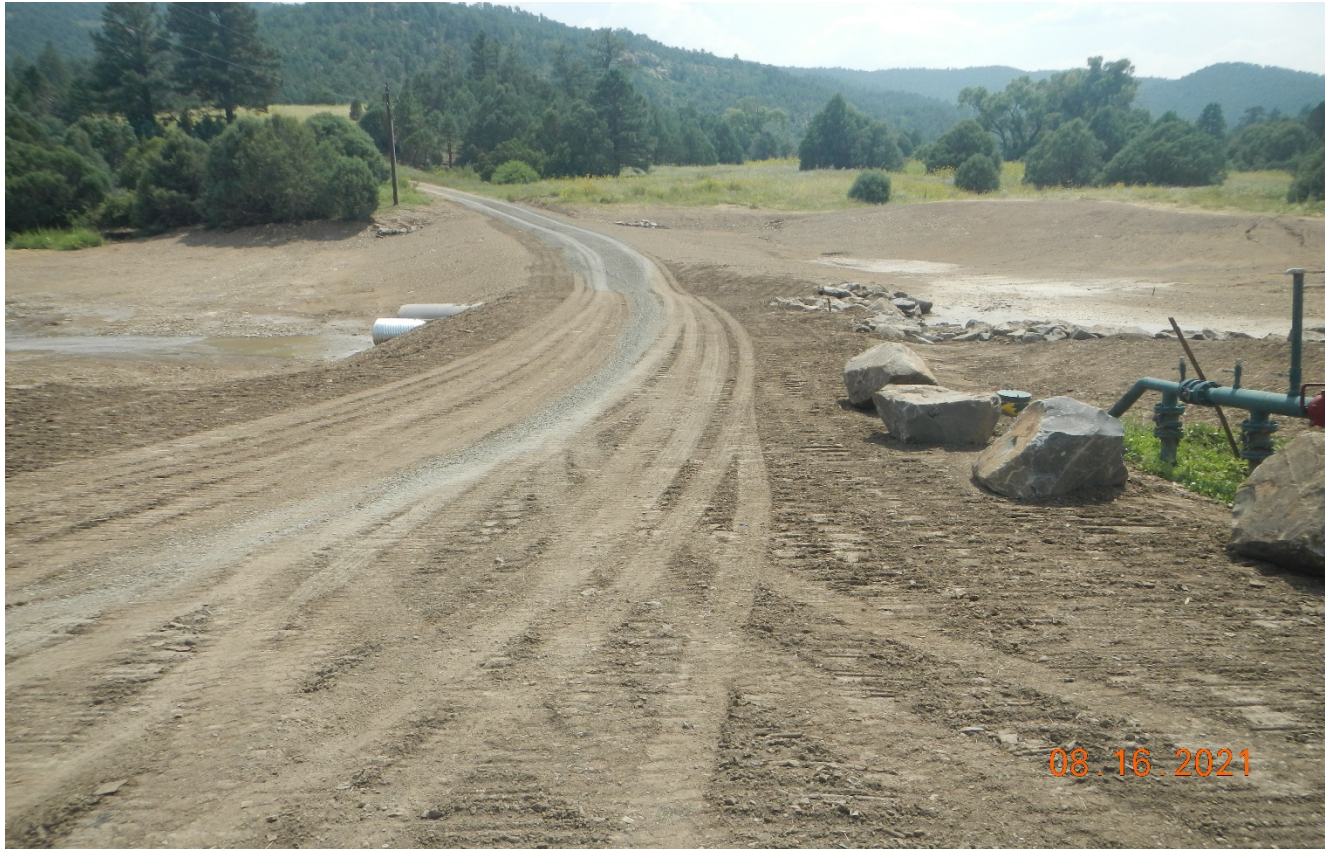
Photo 1. Facing south toward the access road stream crossing which was washed out during the flood event.
