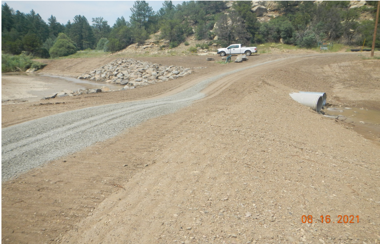
Photo 3. Facing northwest at the stream crossing. There is no bank stabilization at the outlet side.
