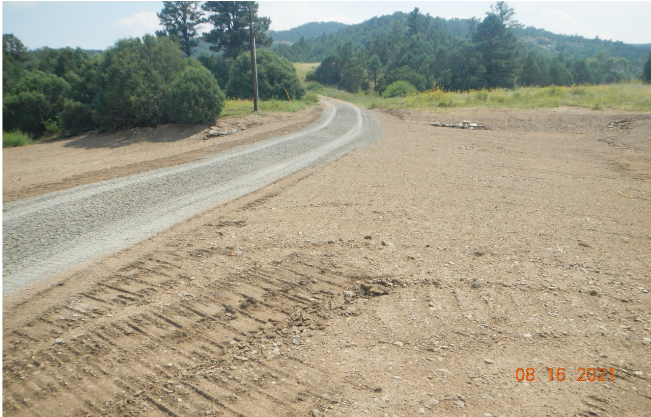
Photo 4. Facing southeast along the access road. Gravel was being hauled to the road during inspection. All disturbed areas will need to be seeded and stabilized.
