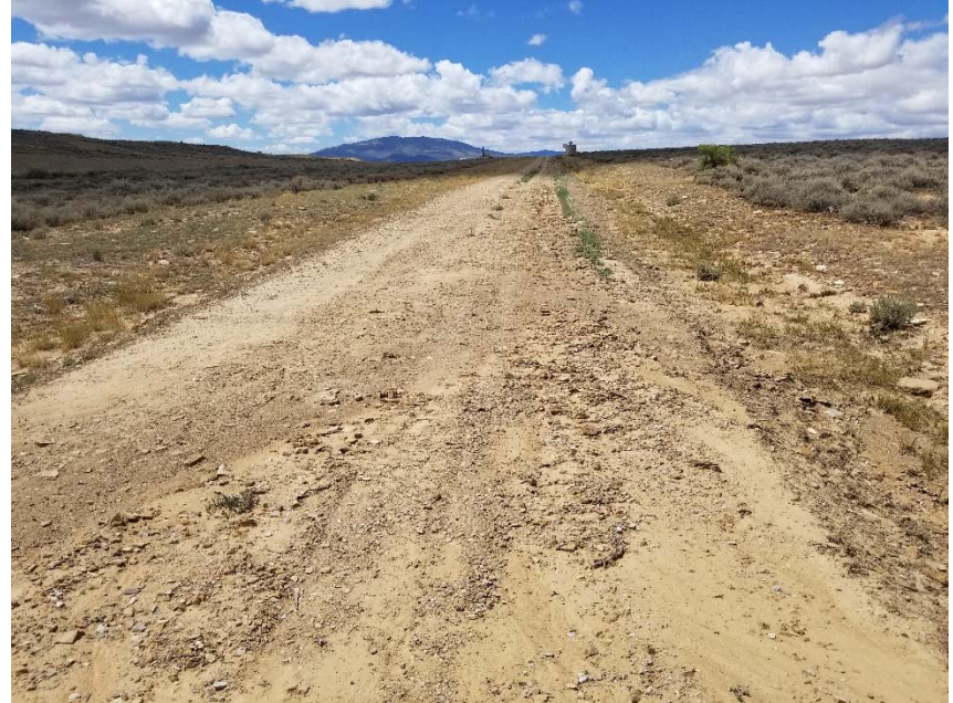
Photo 2. Sediment migration onto and across access road.
