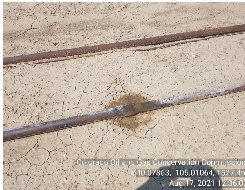
Photo 4 Stained soil and mechanical issue 2" piping to separator.
