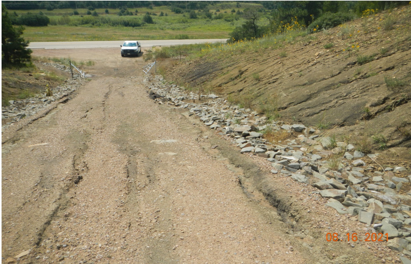
Photo 2. Stormwater is causing erosion down the access road which is filling in the cattleguard. Storm water needs to be diverted off the road to prevent erosion (berm, water bar). The cut slopes shown in upper right of the photo are not stabilized.
