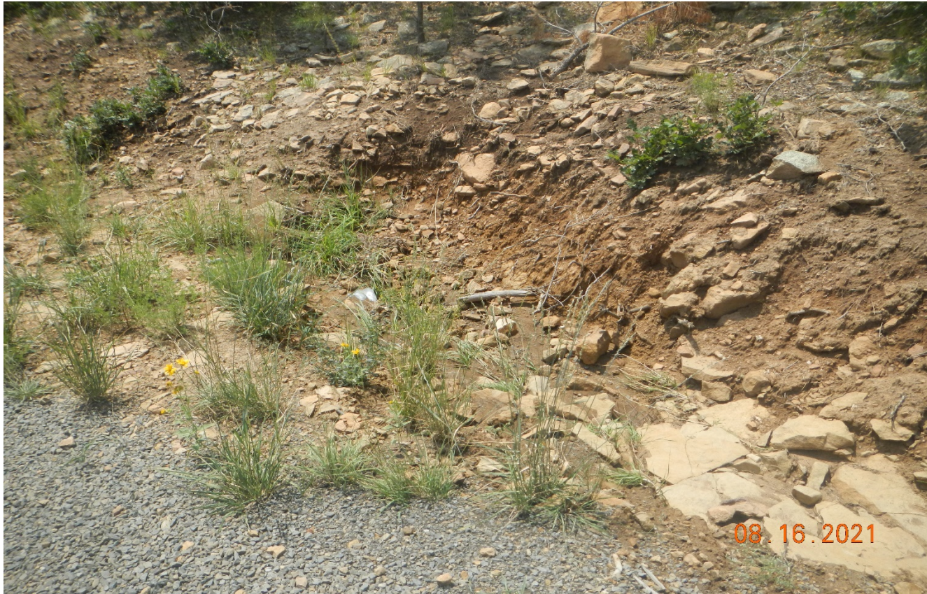
Photo 4. Sediment has accumulated in this culvert along the road.
