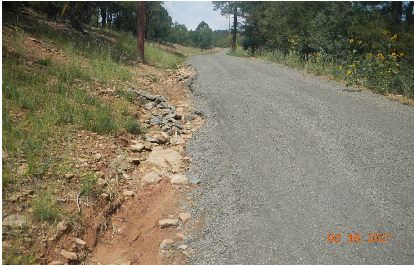
Photo 3. Facing west along the access road. The rock check dam has washed out and needs repair.
