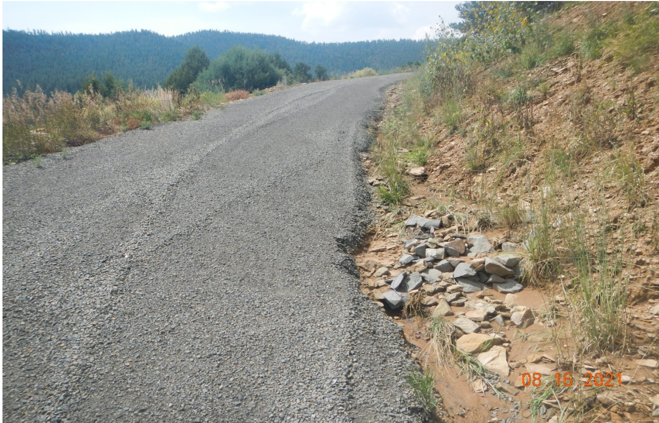
Photo 1. Facing southwest along the access road. The rock check dam has washed out and needs repair.
