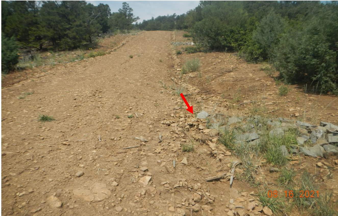
Photo 5. Facing northwest. Stormwater has eroded around the edge of this rock diversion. Additionally the road sides should be seeded to establish vegetation.
