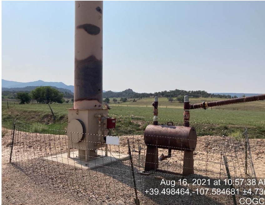
ECD is disconnected (unused equipment)
