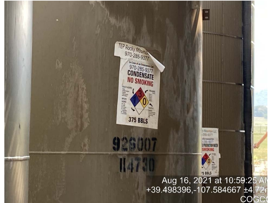
Tank label falling off
