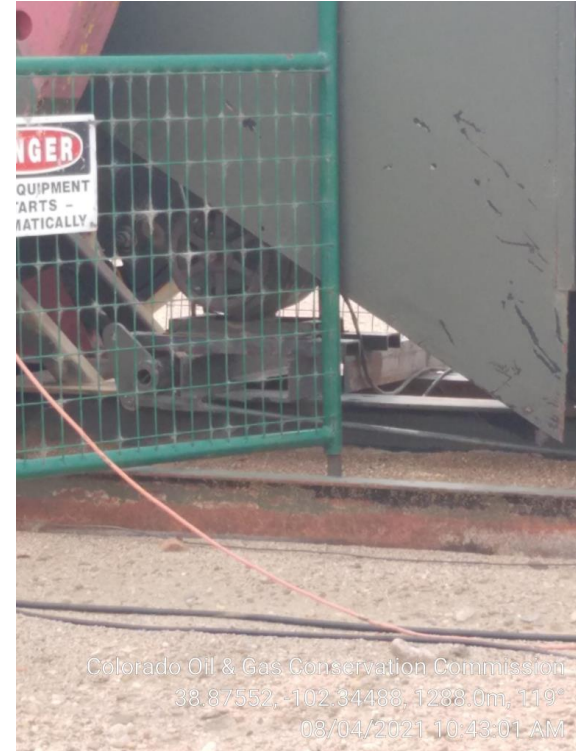
6. Cathodic Generator (Not used)
