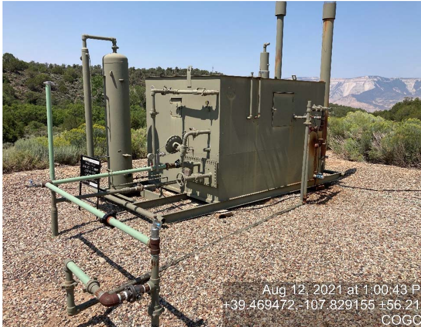
Location/lack of separator bath signage
