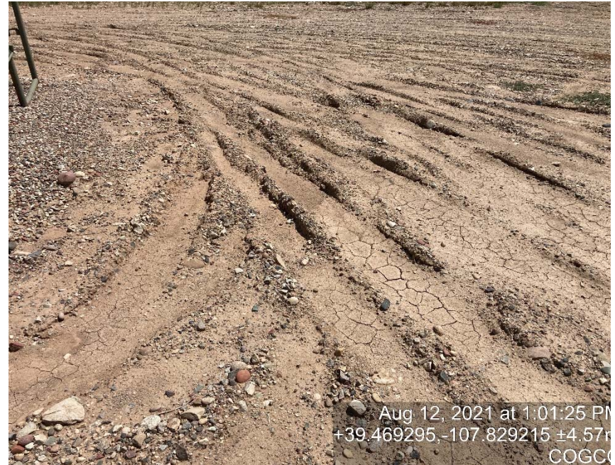
Lack of stabilization/compaction
