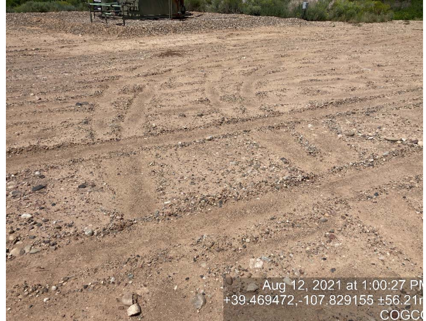
Lack of stabilization/compaction
