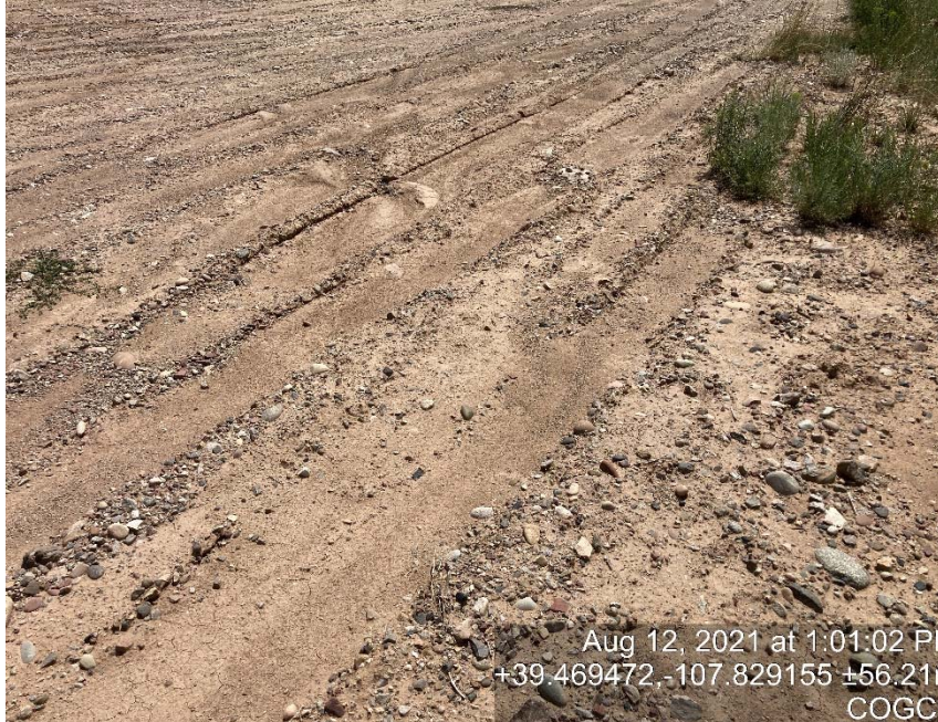
Lack of stabilization/compaction
