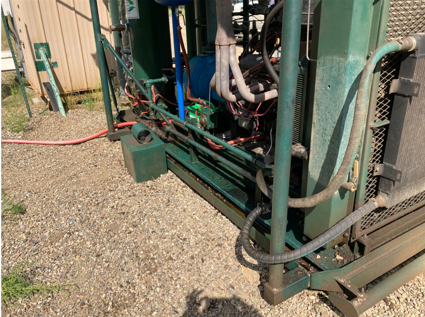
PHOTO 2: ALL VALVES, PIPES AND FITTINGS ARE SECURLY FASTENED. THE OIL ACCUMULATION IN THE RESERVIOR OF THE LIQUID RING SKID WAS REMOVED AND THE IMPACTED SOIL ON THE GROUND WAS CLEANED UP.
