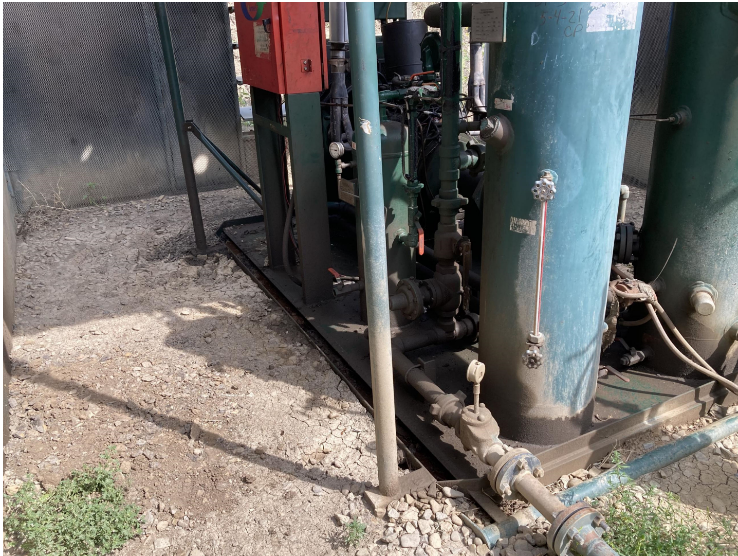
PHOTO 3: THE OIL ACCUMULATION IN THE RESERVIOR OF THE LIQUID RING SKID WAS REMOVED AND THE IMPACTED SOIL NEXT TO THE LIQUID RING COMPRESSOR WAS REMOVED AND PROPERLY DISPOSED IN ACCORDANCE WITH THE OGRIS OPERATING WASTE MANAGEMENT PLAN.
