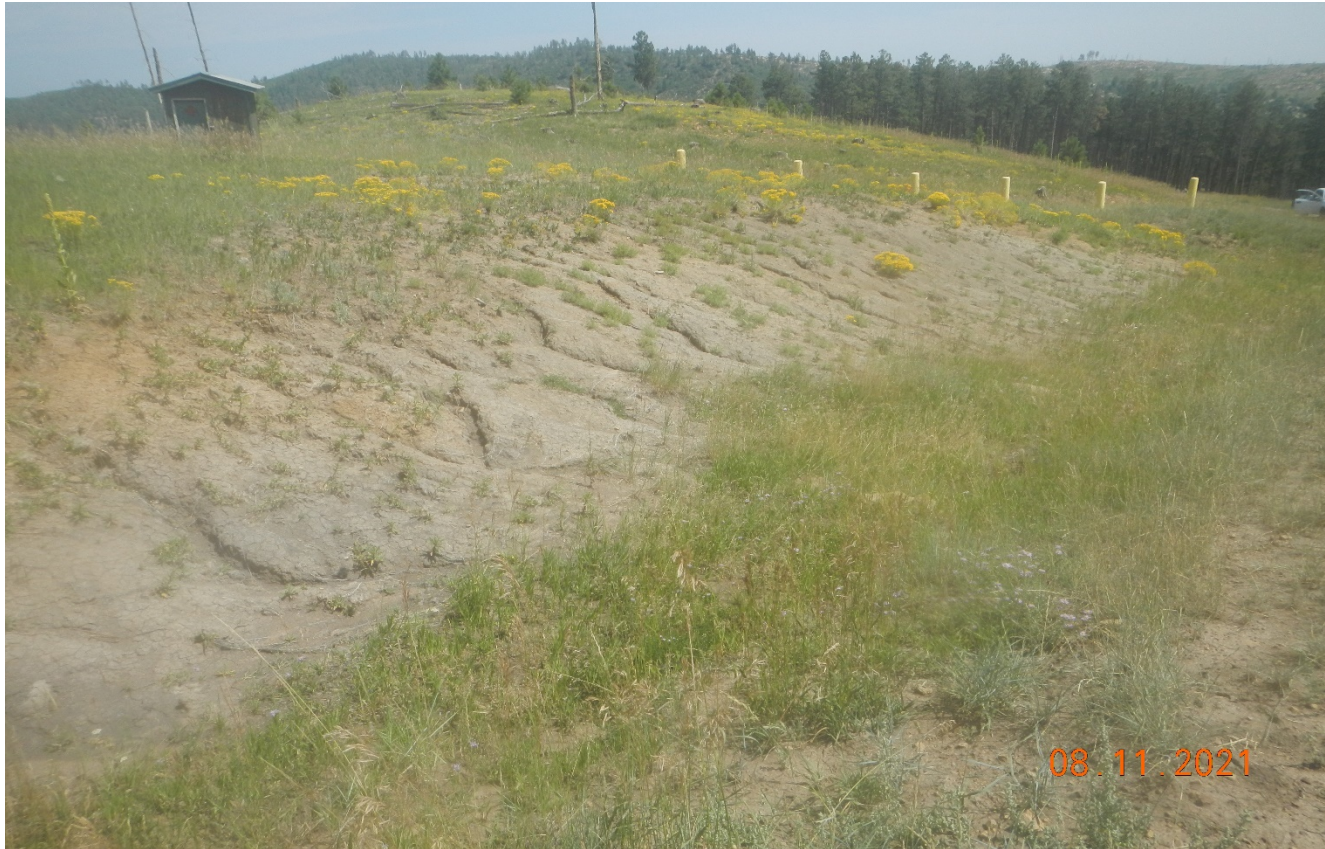
Photo 6. Facing toward the northwest side of the location. This area is not stabilized and additional reclamation will need to be performed in this area.
