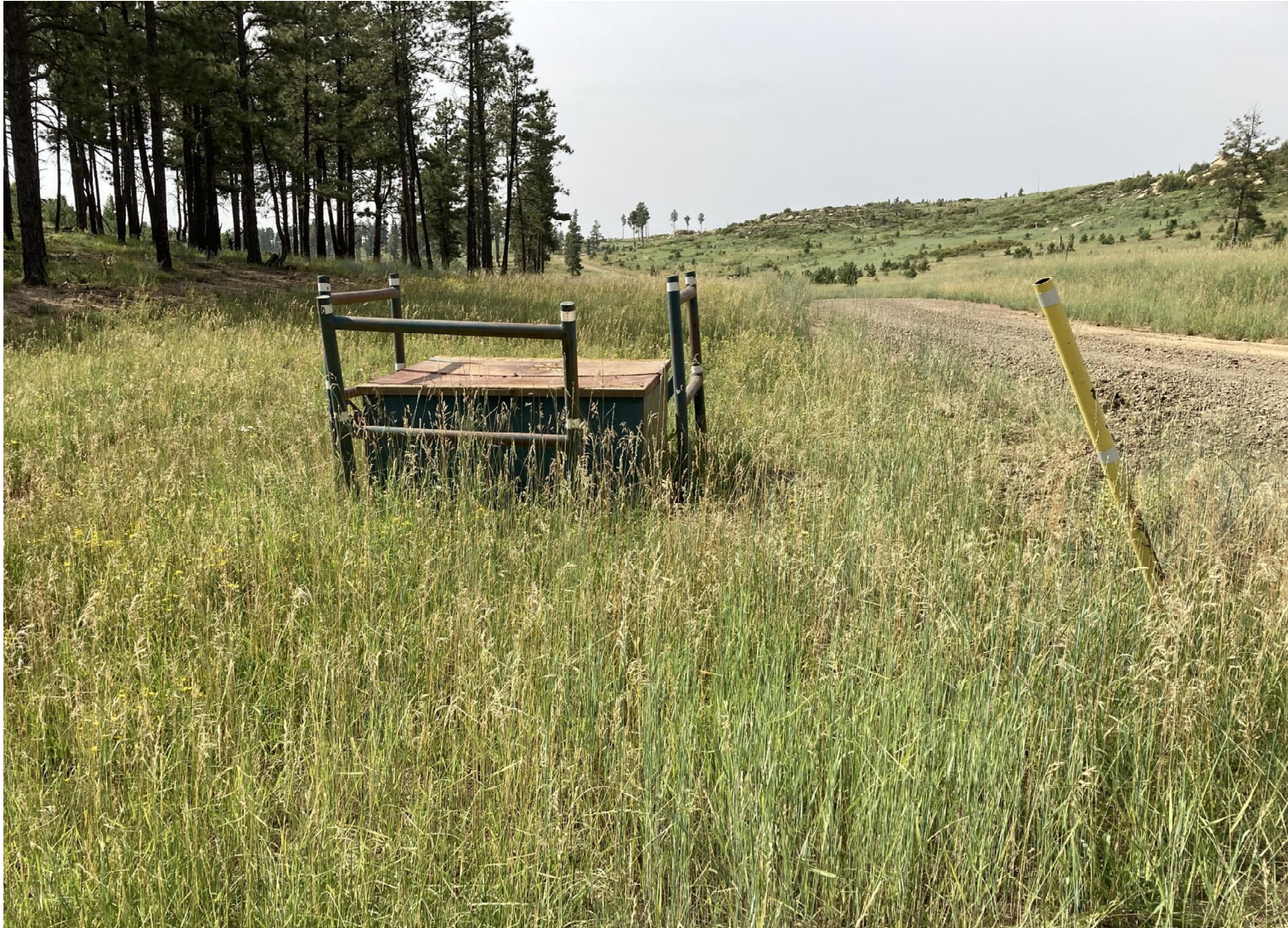
PHOTO 1: THE ORANGE FLAGGER TAPE WAS REMOVED. THIS WAS USED TO MARK THE END OF THE LEASE RUN FOR NEW HIRES. THERE WERE NO PIPELINE ISSUES, SOMEONE UNCOVERED THE VALVE CAN TO SEE WHAT WAS INSIDE AND FAILED TO REPLACE THE LID AS IT WAS TOO HEAVY. THE VALVE CAN COVER WAS PLACED BACK ON TOP OF THE VALVE CAN.
