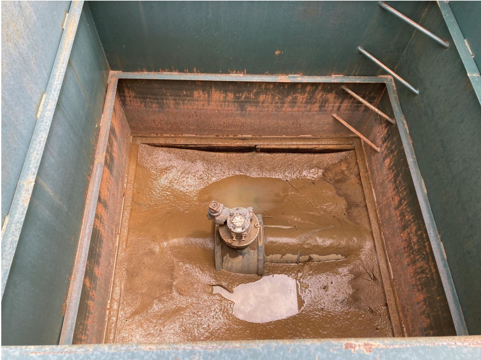
PHOTO 2: THE PIPELINE VALVE IS IN GOOD MECHANICAL CONDITION, THERE WERE NO ISSUES WITH THE PIPELINE. THE WATER IN THE VALVE BOX WAS RAIN WATER ONLY. THE ORANGE FLAGGER TAPE THAT WAS USED AT THIS INTERSECTION TO INDICATE THE END OF THAT RUN FOR NEW EMPLOYEE'S/CONTRACTOR'S HAS BEEN REMOVED.
