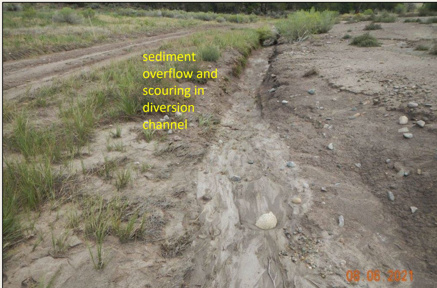
Photo 4. View of erosional down-cutting and sediment discharge within the northern well pad diversion.
