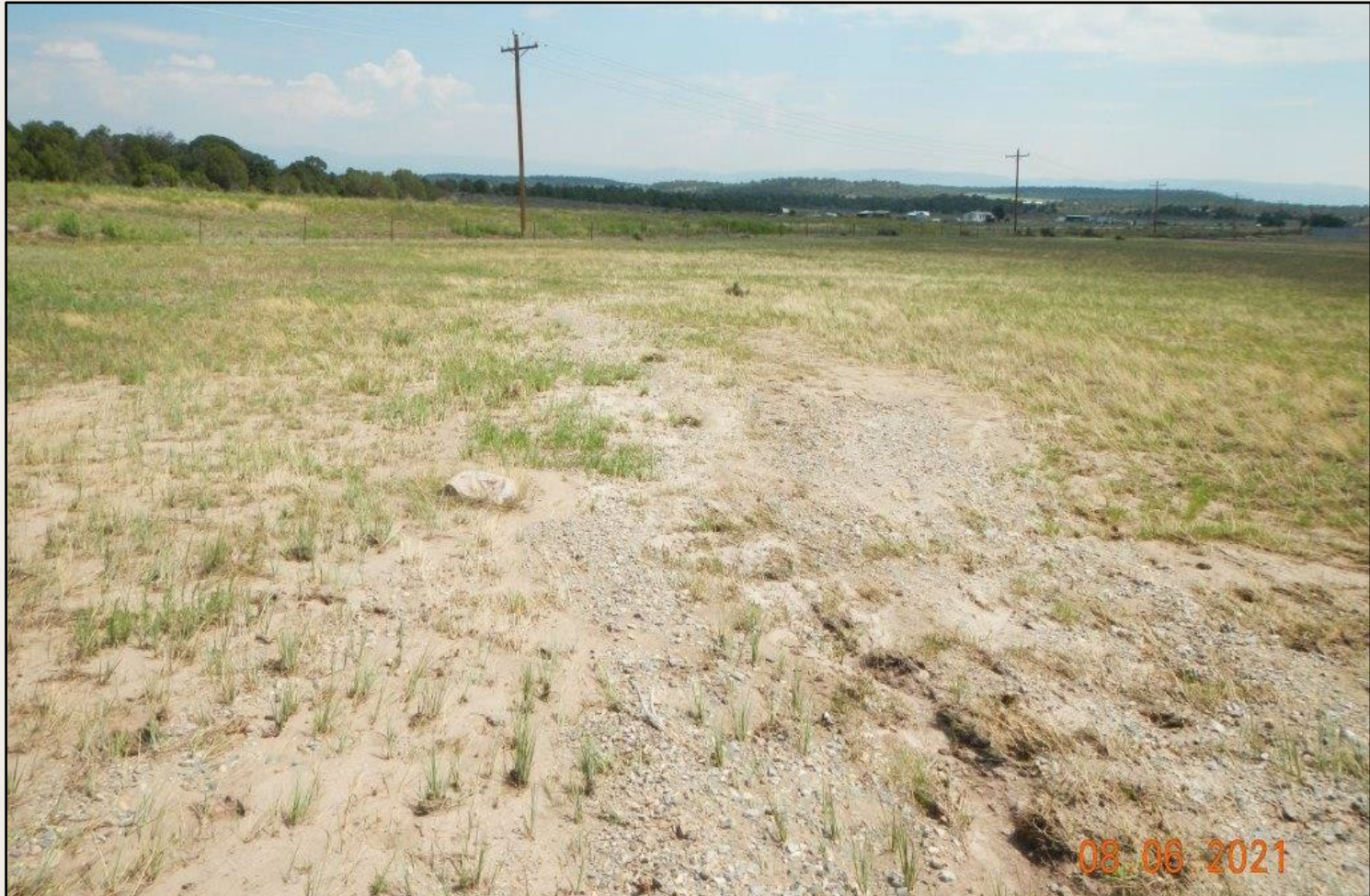
Photo 9. View of discharged sediment and gravel, as well as an erosional feature forming down-slope of Photo 8, facing downstream. Gravel and excess material needs to be removed and area needs revegetation.
