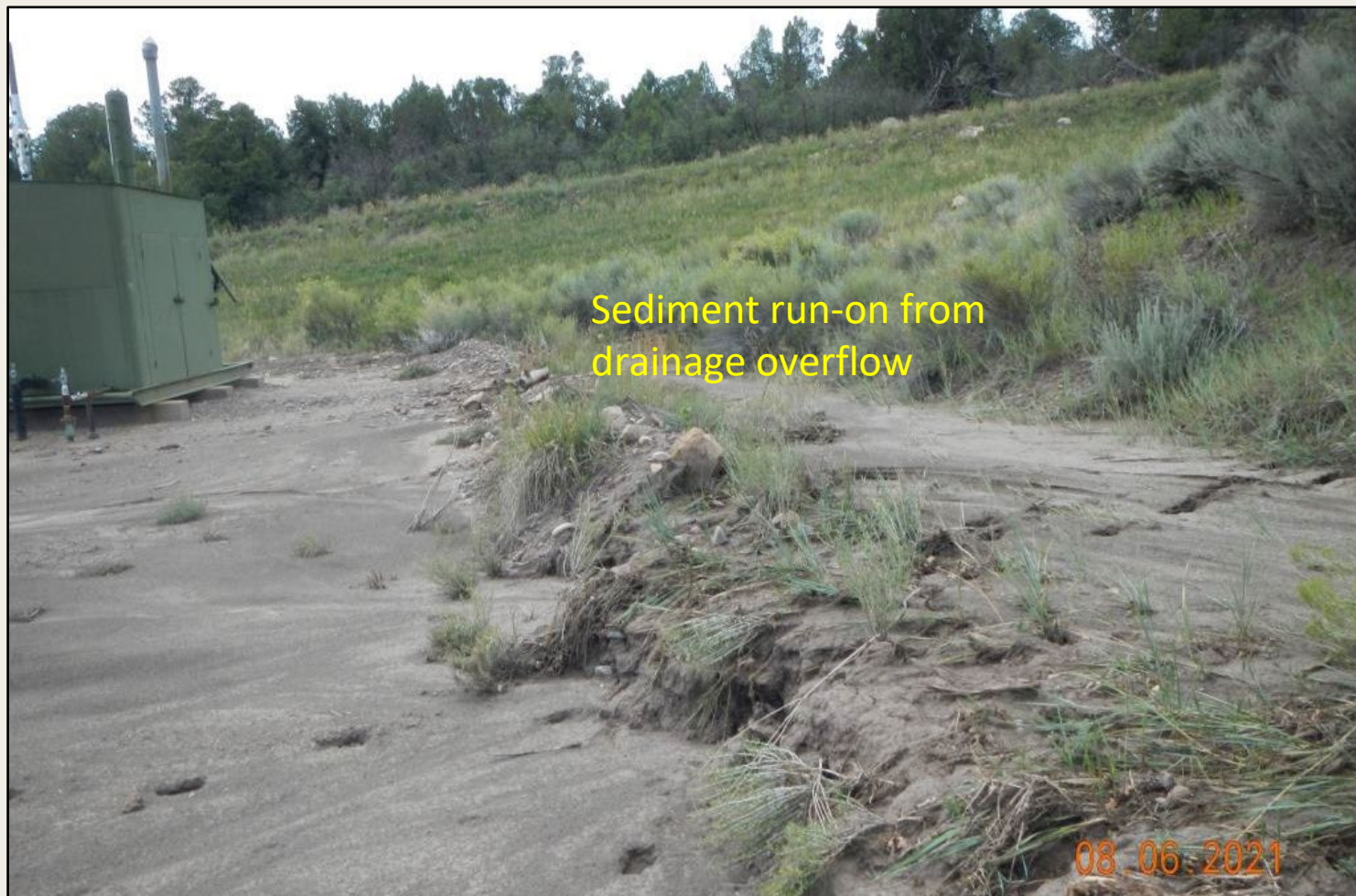
Photo 3. View of sediment discharge and run-on from overflowing in the northwestern stormwater diversion.
