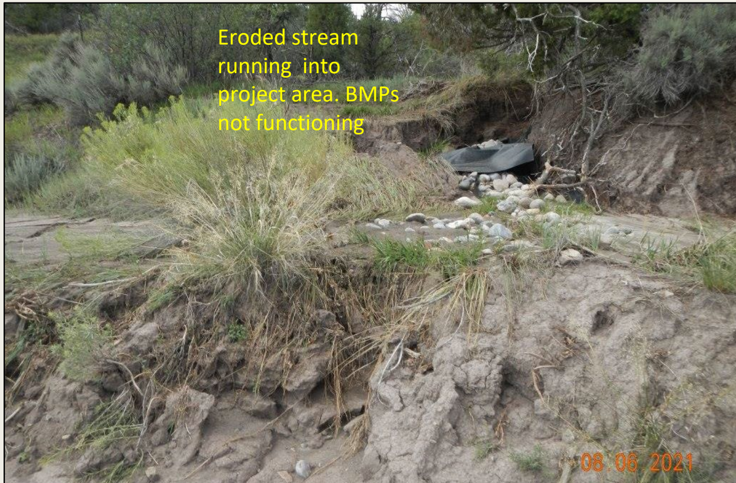
Photo 2. View of erosional headcutting and sediment deposition due to failed BMPs within the western project area.
