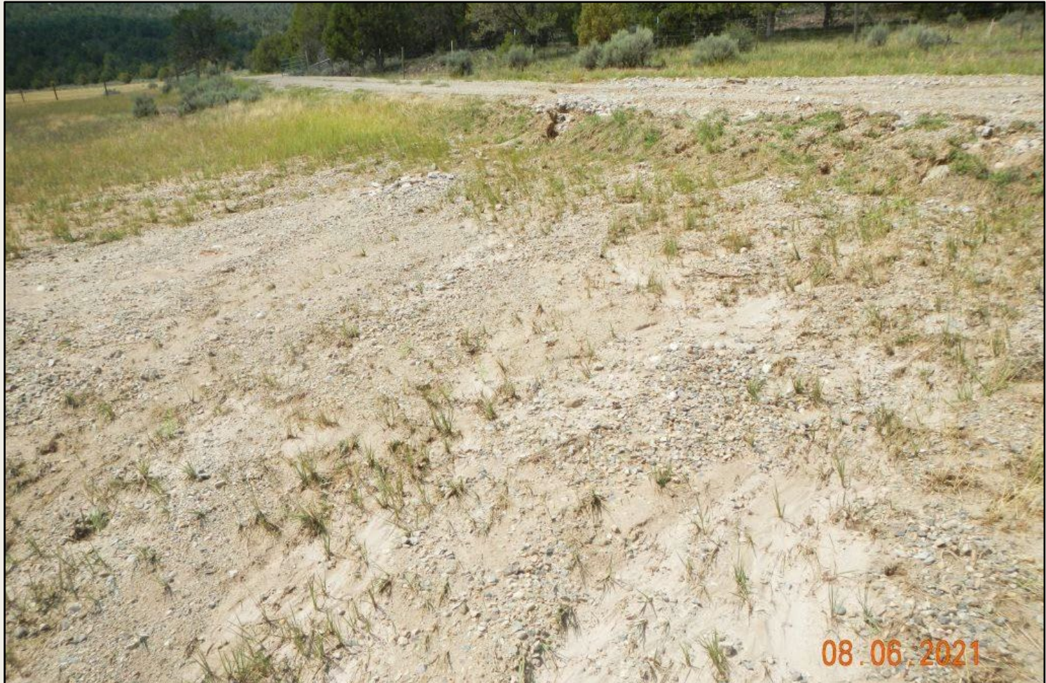
Photo 8. View of another portion of the access road (facing up-slope) where stormwater flows have not been properly contained and resulted in overflow and sediment discharge.
