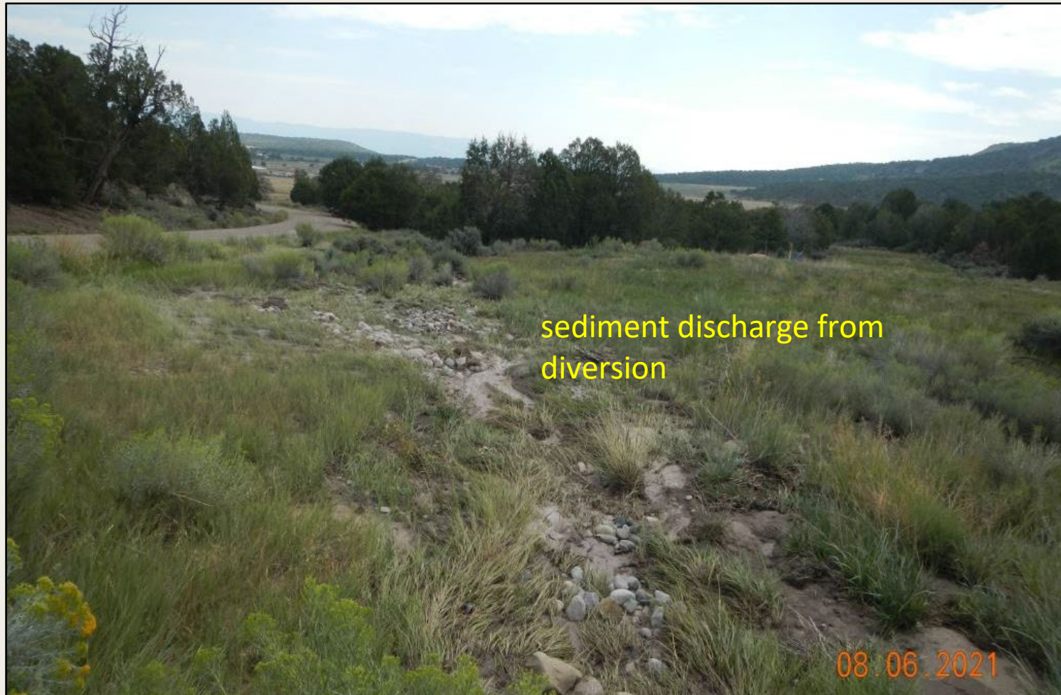
Photo 5. View of rock, gravel, and sediment discharge from the northern well pad diversion. Facing eastward (downslope). Material needs to be removed
