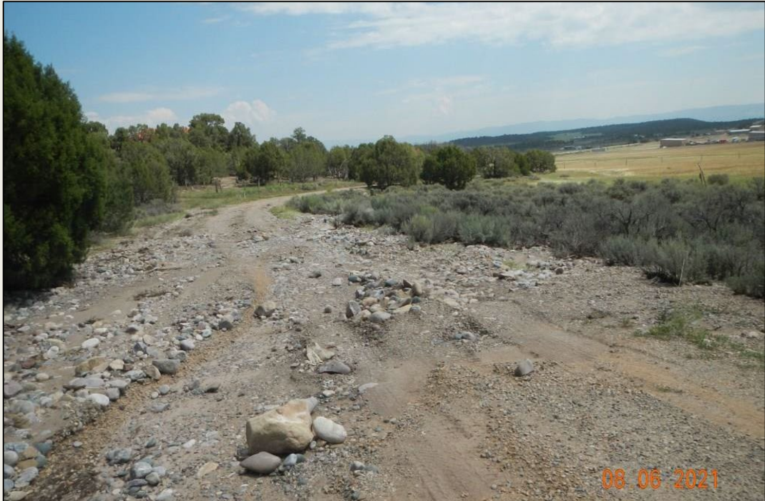
Photo 6. View of area along the access road where stormwater flows have washed out the road.
