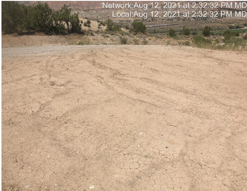
Photo #4797 Insufficient tracking BMP at entrance to location.
