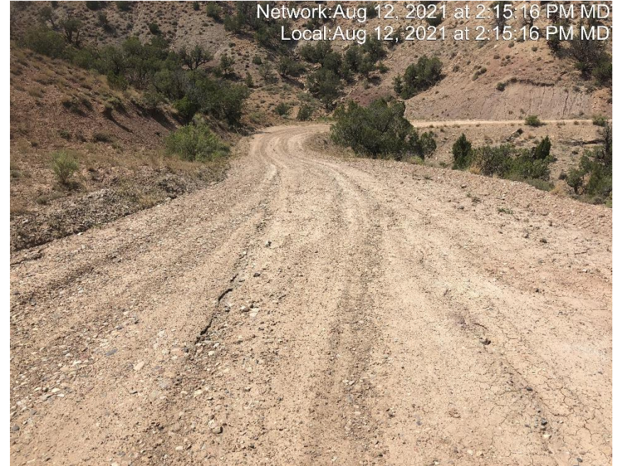
Photo #4789 Insufficient tracking BMP at entrance to location.
