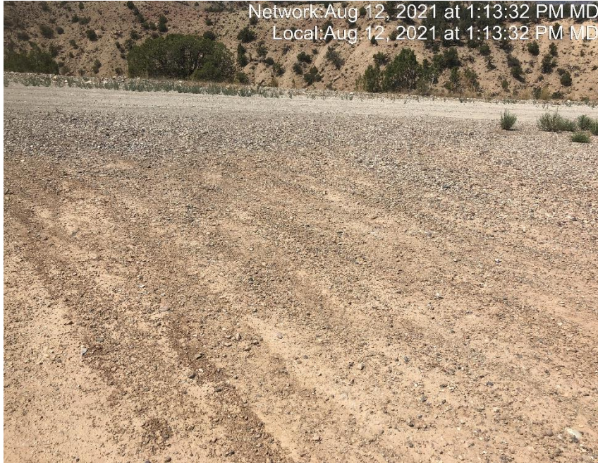
Photo #4785 Insufficient tracking BMP at entrance to location.
