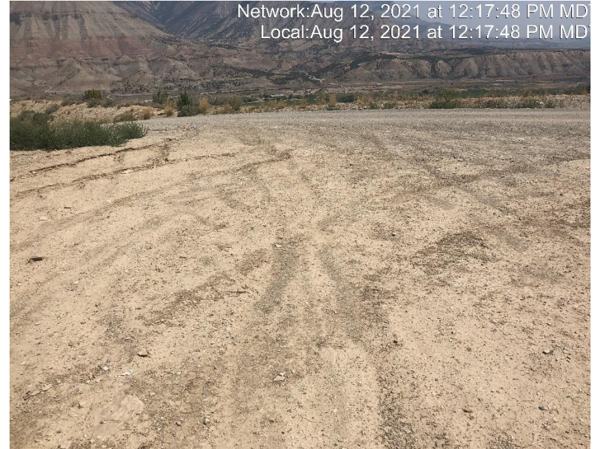
Photo #4780 Insufficient tracking BMP at entrance to location.
