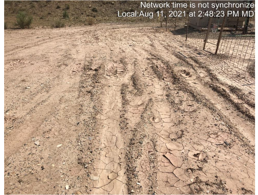
Photo #4768 Location lacks stabilization.
