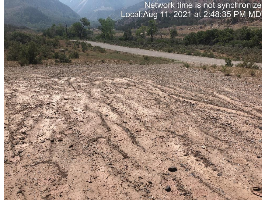
Photo #4771 Insufficient tracking controls at entrance to location.
