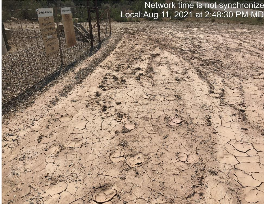
Photo #4770 Location lacks stabilization.
