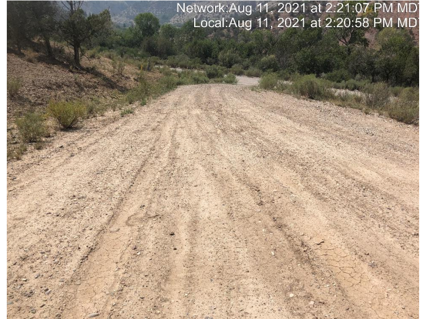
Photo #4764 Insufficient tracking control at entrance to location.
