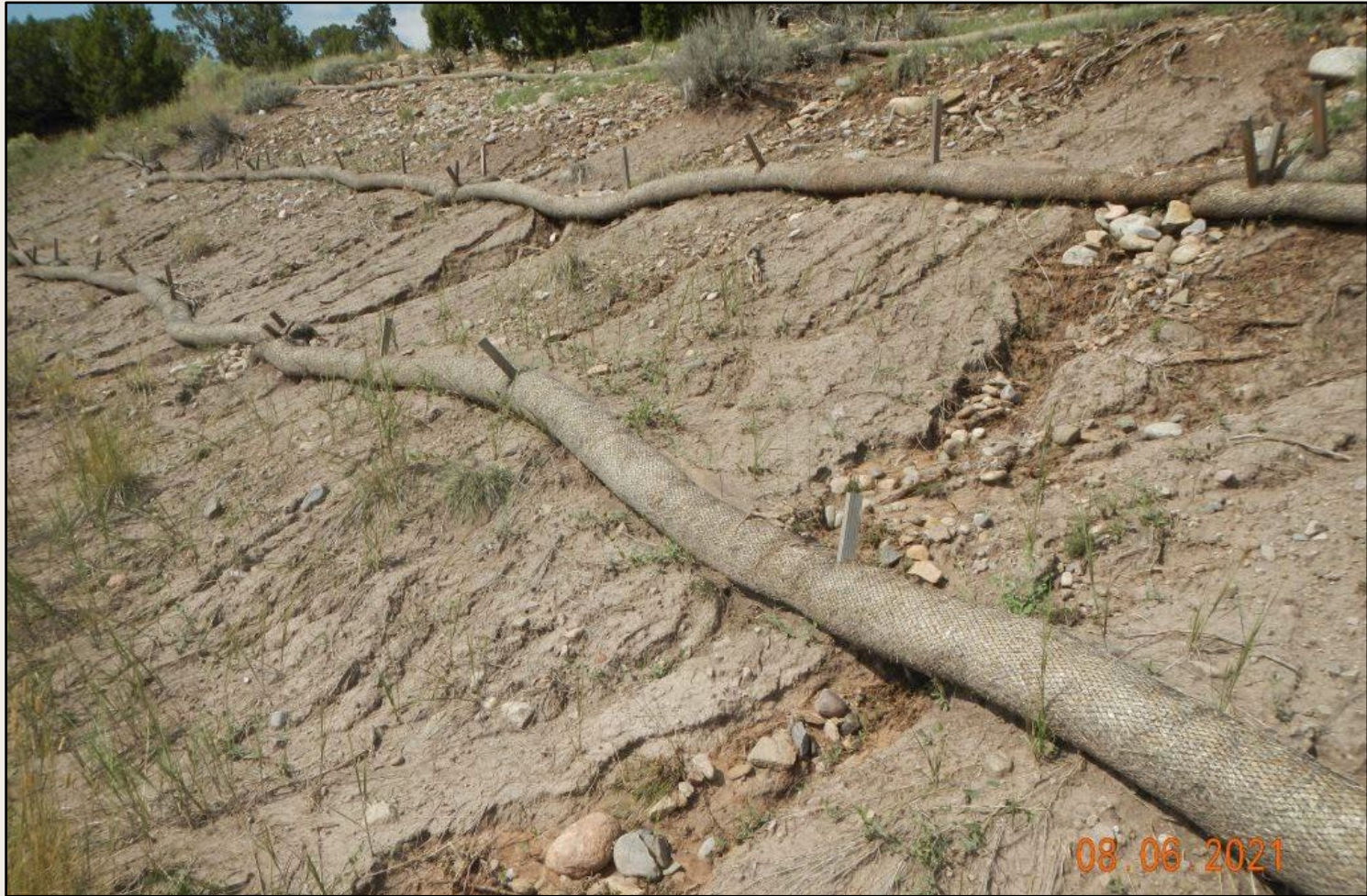
Photo 3. View of failed wattles and erosion occurring on the well pad cut-slope. Wattles are not an adequate BMP here. Long term stabilization measures are needed until stabilized with desirable perennial vegetation.
