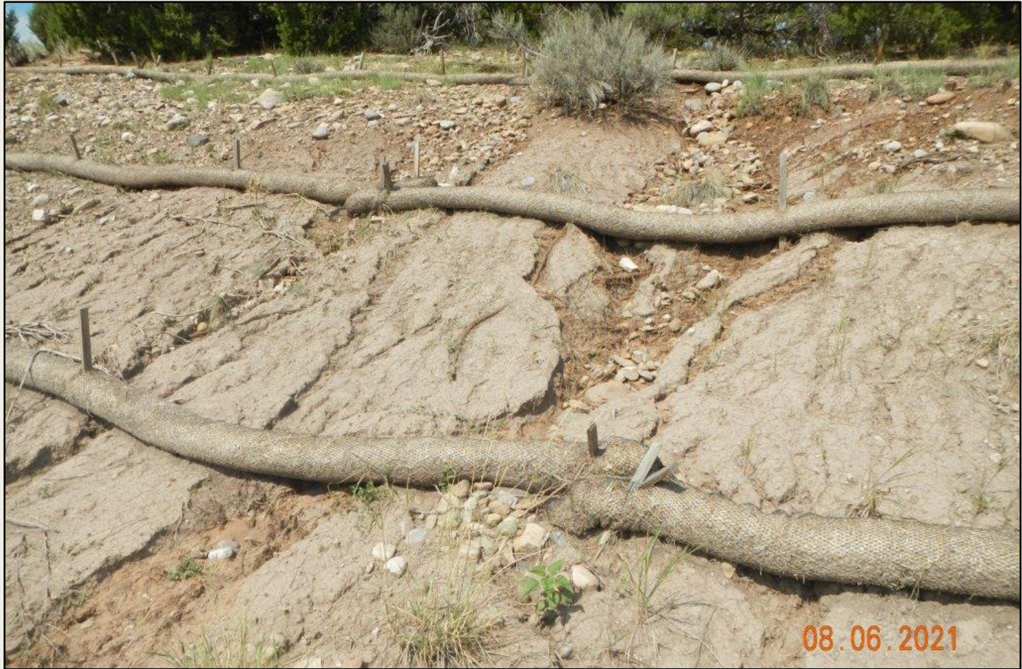
Photo 4. Another view of erosional channeling and failure of wattles on well pad cut-slope.
